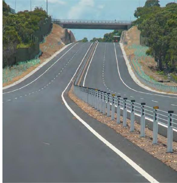
The function of the Bangor Bypass as a major arterial road is clear. While drivers would feel comfortable travelling at certain speeds, the particular sight distances and setbacks would make motorway type speeds feel uncomfortable. The whole project has been designed to clearly give the appearance of a major road.
