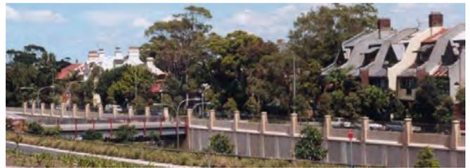
The depressed motorway is hidden from the houses and park. Its retaining walls minimise its footprint and are designed to complement the form of the Victorian terraced houses of Surry Hills.
