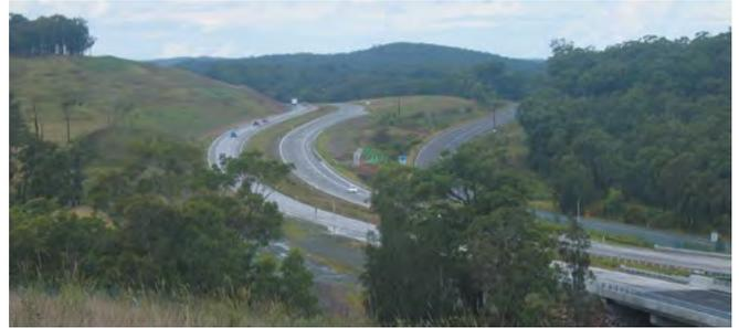
Karuah to Bulahdelah: Rounding off and grading out the slopes to 1:4 create an almost seamless integration with the natural slopes.
