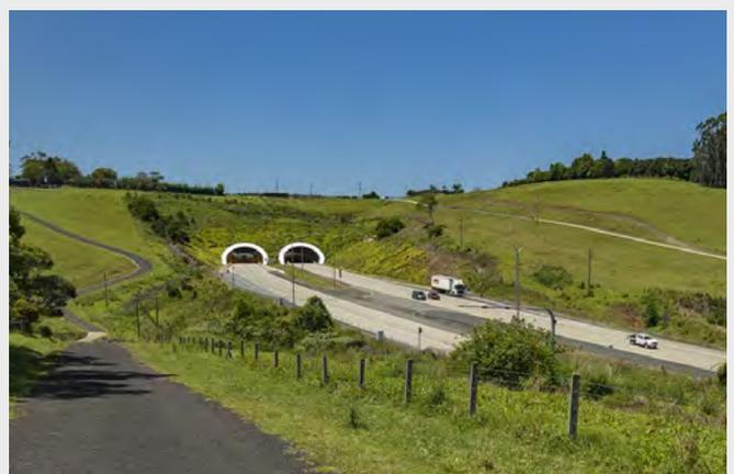
The white tunnel portal collars contrast and highlight the landscape and landform around. They divert storm water and provide a maintenance safety parapet. The landform wrapped around the portals and laid back to natural grades is a long term safe earthworks solution which avoids walls, their maintenance and graffiti.
