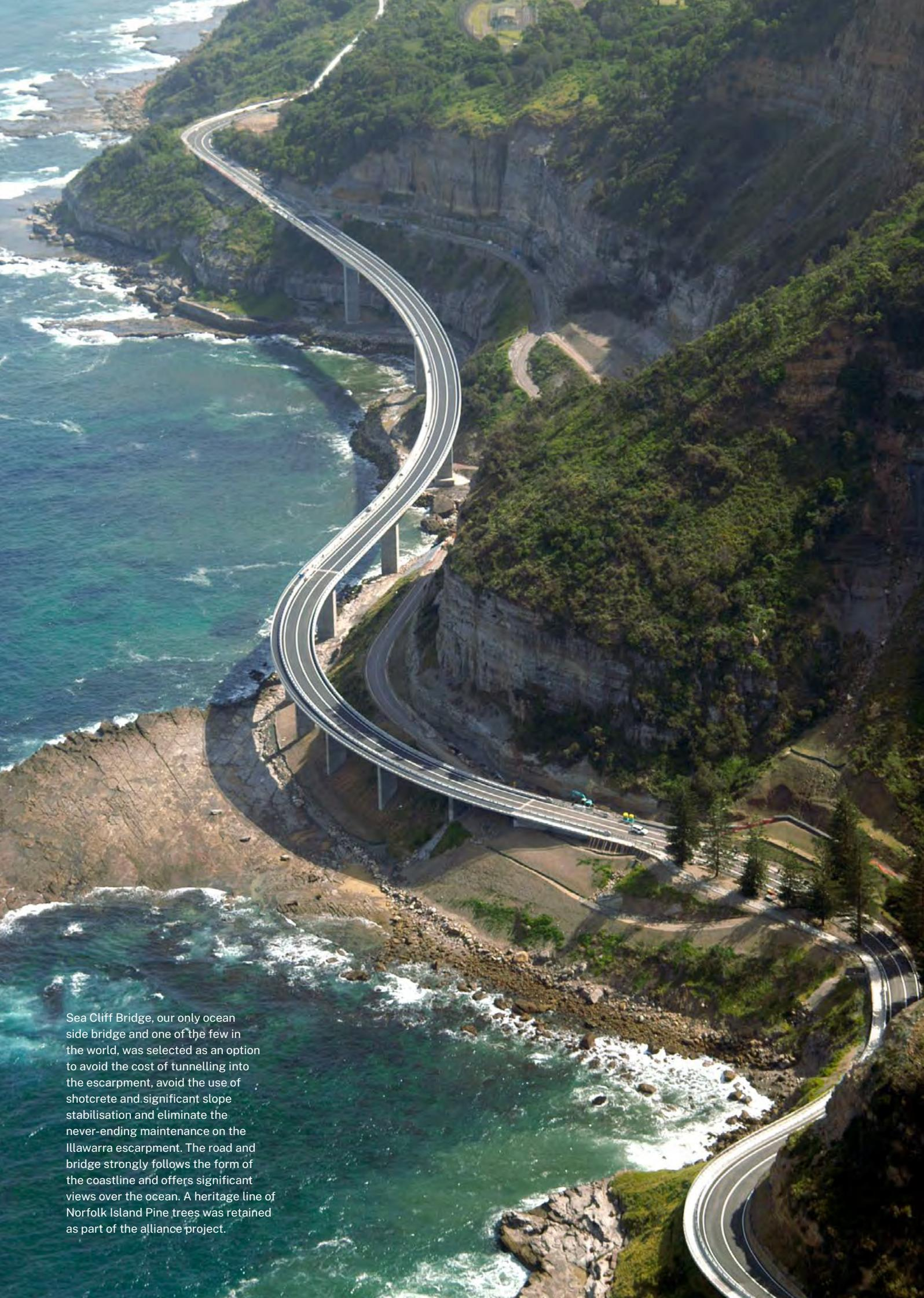
Sea Cliff Bridge, our only ocean side bridge and one of the few in the world, was selected as an option to avoid the cost of tunnelling into the escarpment, avoid the use of shotcrete and significant slope stabilisation and eliminate the never-ending maintenance on the Illawarra escarpment. The road and bridge strongly follows the form of the coastline and offers significant views over the ocean. A heritage line of Norfolk Island Pine trees was retained as part of the alliance project.
