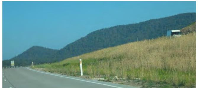
Karuah Bypass: Independently grading the carriageways helps minimise earthworks, provides a more interesting journey and reduces the wide terraced effect of roads on hillsides. Note the gentle gradient of the embankment.
