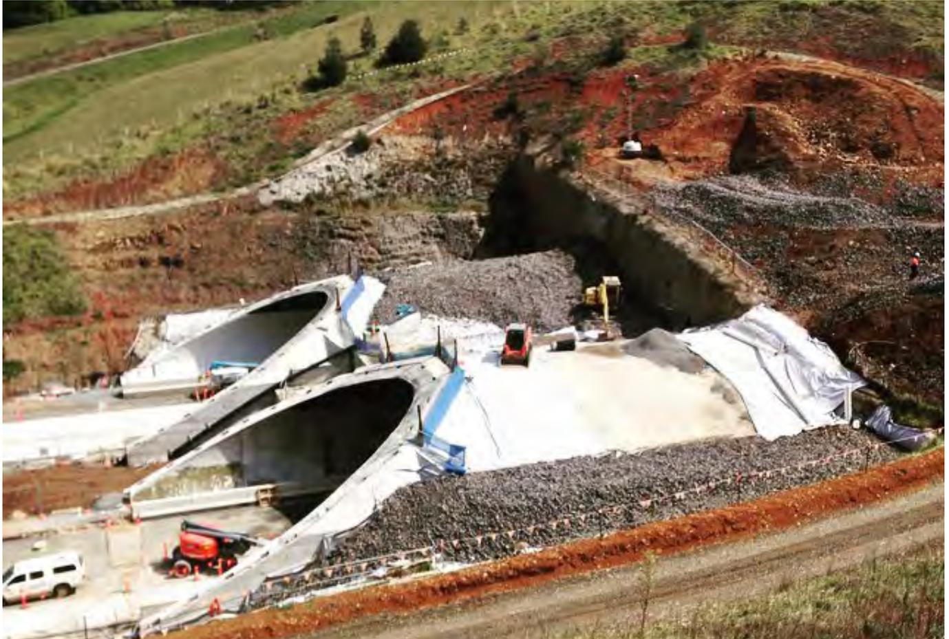
The design needs monitoring during construction. Checking earthworks shaping, signing off on trial panels, ad hoc advice on design changes, and planting operations oversight are all important aspects of ensuring a project turns out well. In this example on the Tintenbar to Ewingsdale tunnel the monitoring was important to check that the landform wrapping around the cut and cover portals was successful.
