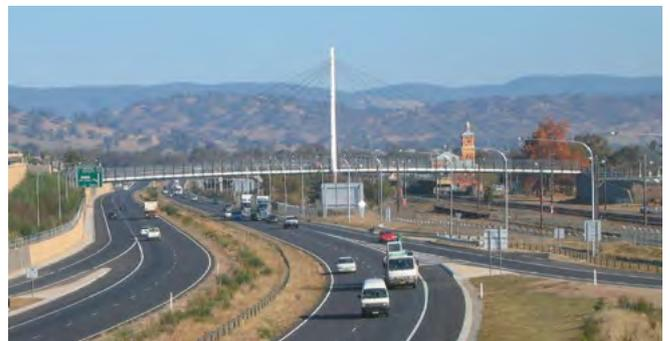
The approach from the north with the Dean Street cable-stay pedestrian bridge and old railway station and yards in view. The terraced retaining walls and noise walls align with the town grid and complement the station.
