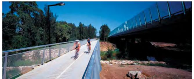
The design of the 40 kilometre shared path is unified with the rest of the project and built with durable materials such as this concrete decking over a creek.
