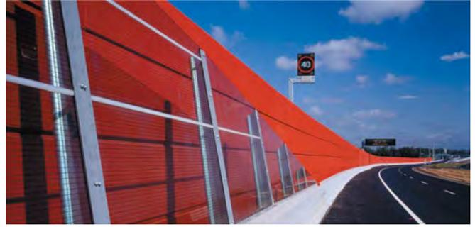
Clear walls always overlap solid walls and primary colours are used to emphasise different character zones along the M7 Motorway. Experience is showing that laminated and toughened glass would be best substituted by transparent plastic products in future.
