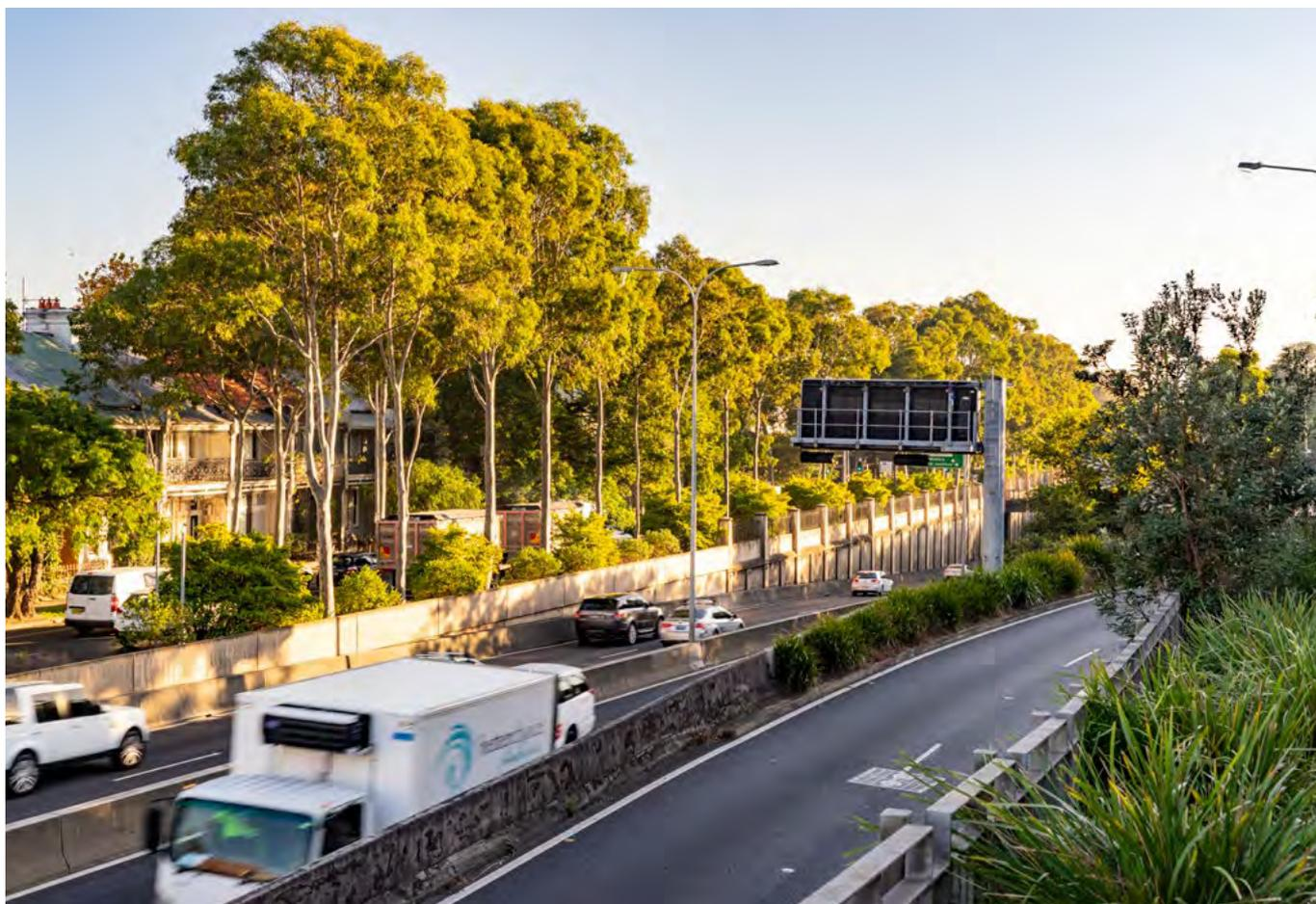
The Eastern Distributor was set down into a trench, minimising visual and noise impacts. Retaining walls ensured a minimal footprint and were designed to respond to the Victorian Terrace architecture on South Dowling Street.
