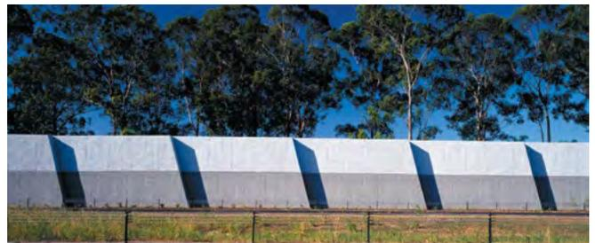
Precast concrete noise walls are designed to serve different purposes and suit different locations. These panels, at a location close to the road, are repetitive and easy to replace. Overpainting is carried out in the event of graffiti vandalism.
