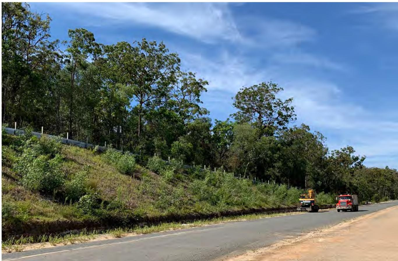
Progressive landscape completion on the Woolgoolga to Ballina section of the Pacific Highway upgrade. The slope gradient, the substrate roughness, the soil depths, the use of locally won soils and the native seeding have all contributed to an outcome that, with appropriate establishment, will provide a long term landscape for the motorway. Creating this outcome progressively helps minimise erosion of uncovered surfaces and helps provide a green outcome on opening.
