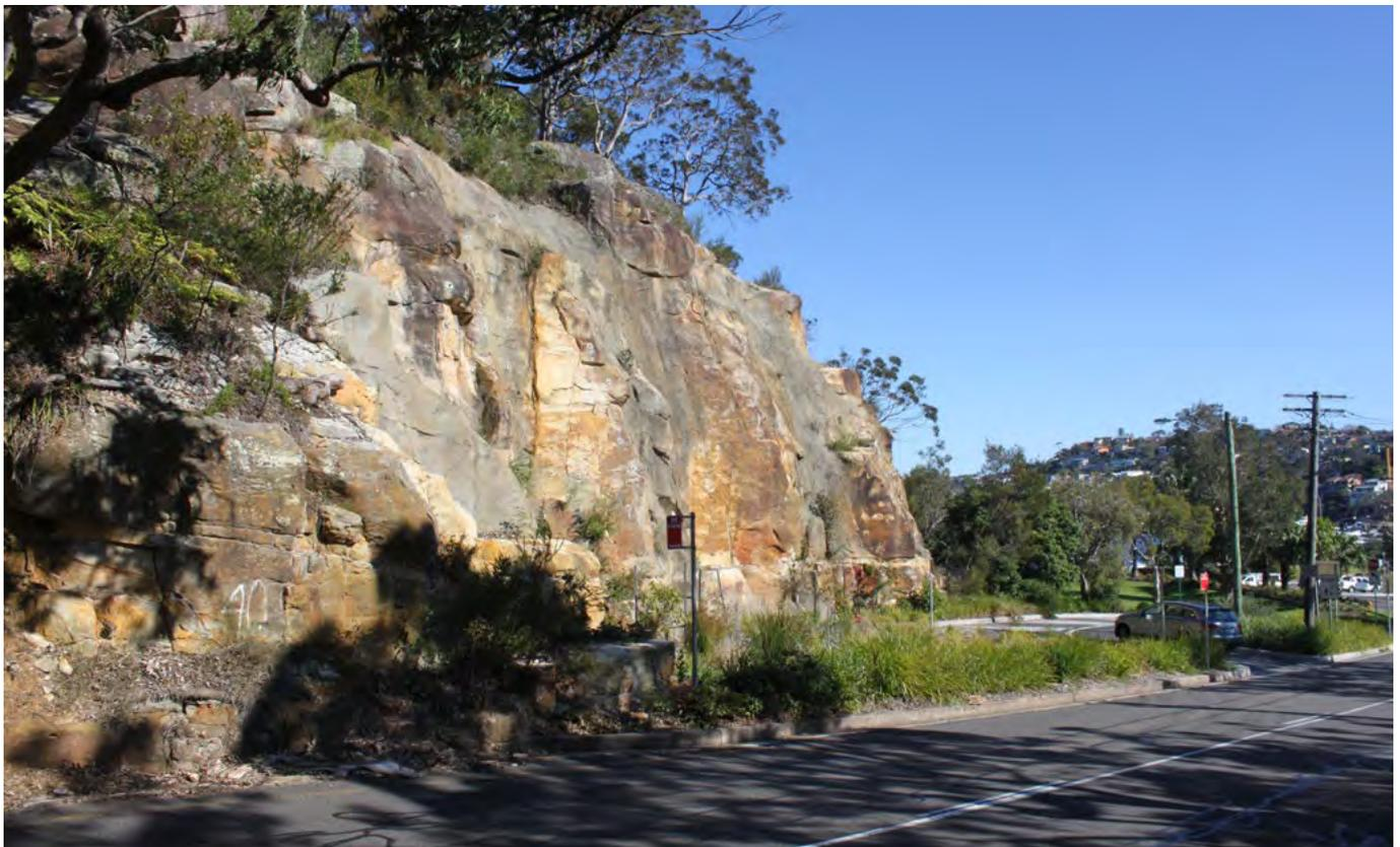
A combination of stable rock with a textured shotcrete applied in minimal areas to stabilise the cutting and provide structural support (The Spit, Sydney)
