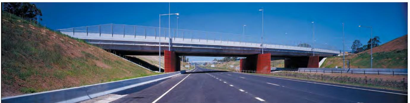
All vehicular bridges have similar properties in terms of coordinated lighting locations, spill-through abutments, tapered safety screens and night lighting. Names of overbridges are neatly integrated with principal designs.
