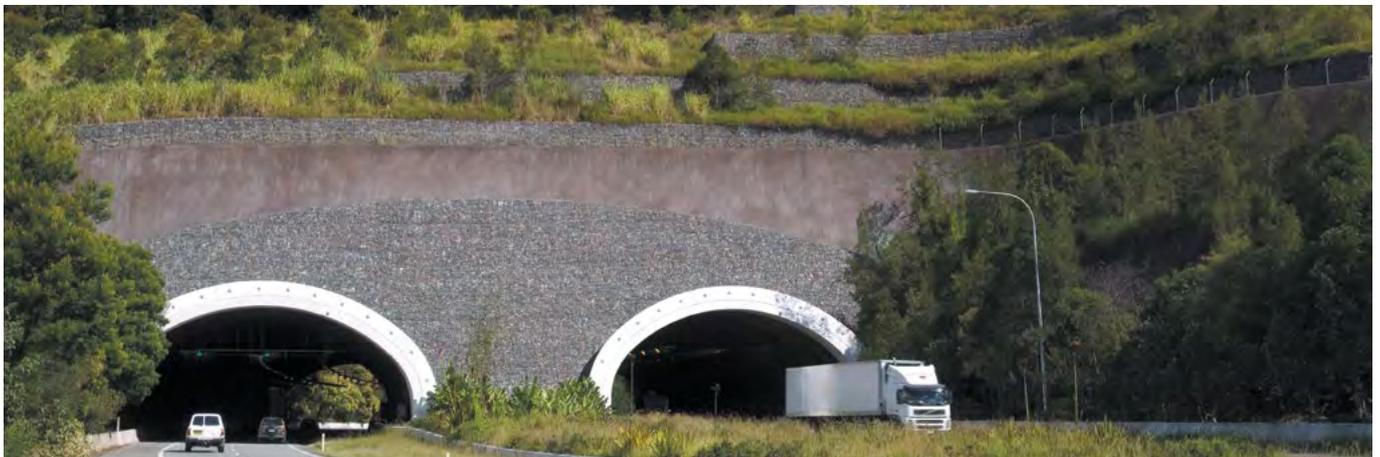
The Cudgen Road tunnel allows the wooded ridge line and wildlife corridor to cross the road and extend down to the edge of the Tweed River. Native planting and seeding is provided to revegetate the edges of the portal. Use of gabion facing is suitable for the natural context.
