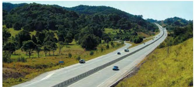
Yelgun to Chinderah: Avoiding cutting through spurs and aiming for saddles and valleys reduces earthworks and creates a more flowing, responsive alignment.
