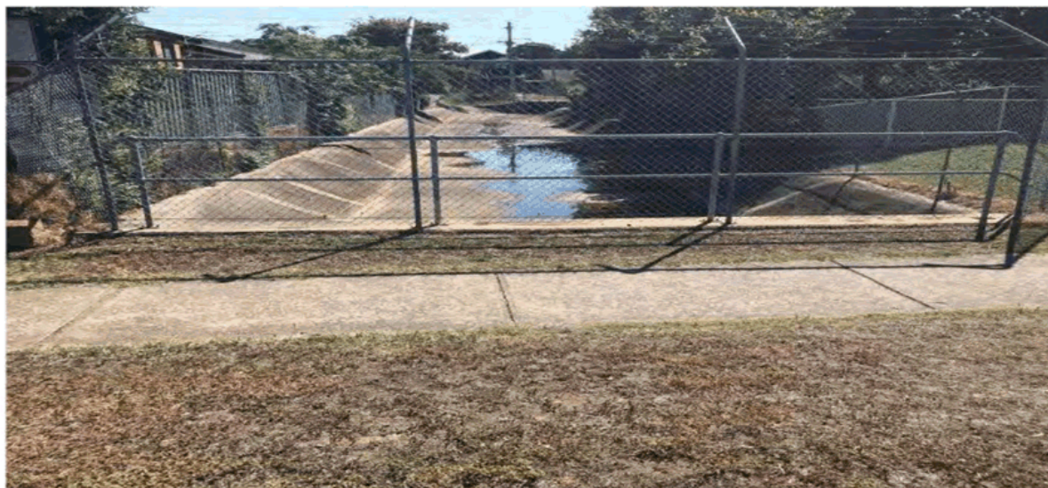
Figure 10: Existing Open Concrete Stormwater Channel Between Cumberland Road and Palmer Street (to be Culverted)
