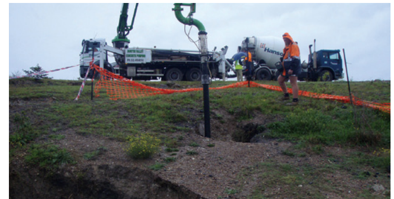
Grouting of pothole at Muswellbrook Common
