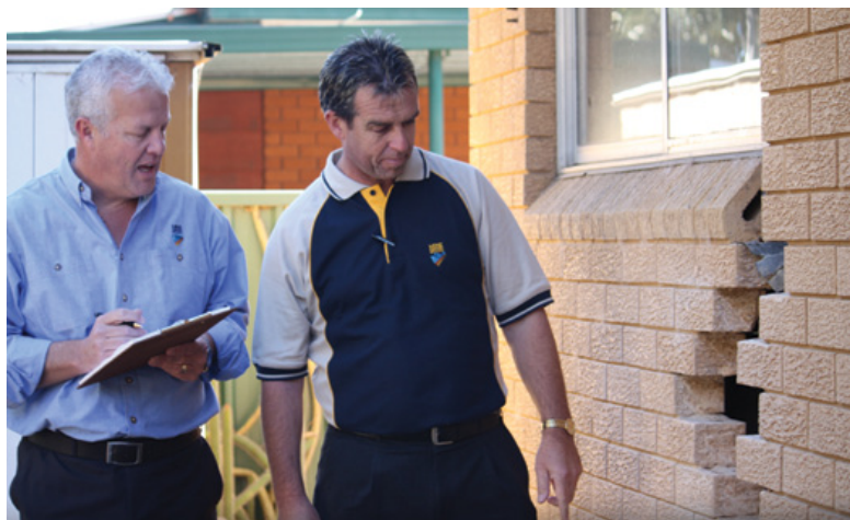
Staff inspecting bricks removed to facilitate the repair of crack in brickwork
