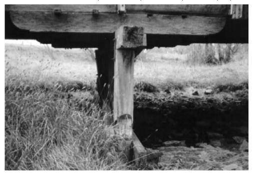
Figure 3.1 Pre-1894 detail of top of trestle of a timber beam bridge
