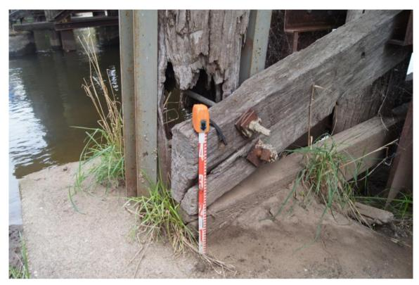
Figure 4.5 Detailed view of decay evident on the base of timber pier support located at the northern end of Towong Bridge
