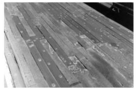
Figure 3.2 First layer of cross planks on the girders shown on the left, while a second layer of longitudinal planks is shown on the right
