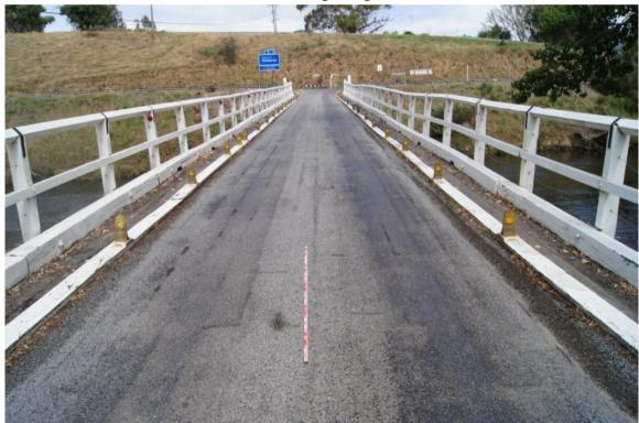
Figure 4.6 Northern approach associated with Towong Bridge showing the bitumen surface of the deck over the original timber decking
