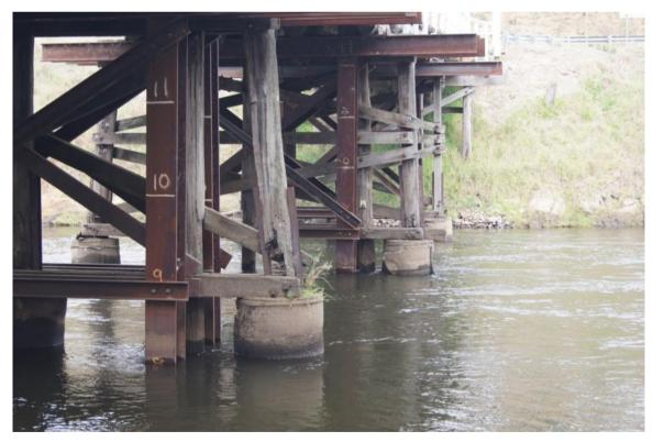
Figure 4.4 North-facing view showing the decay to the base of the timber piers associated with Towong Bridge
