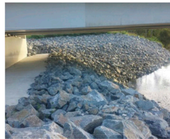
- Rip rap on bridge abutments for scour protection
