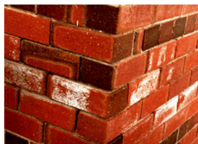
Figure 2.14.1 - Salt damage in the brickwork of buildings identifies a possible salinity problem in the area.
