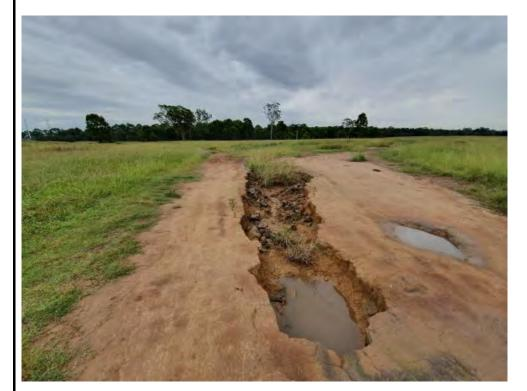
Photograph 16 – Southern Precast Site – Access track washout and dispersive soils (onsite facing east)
