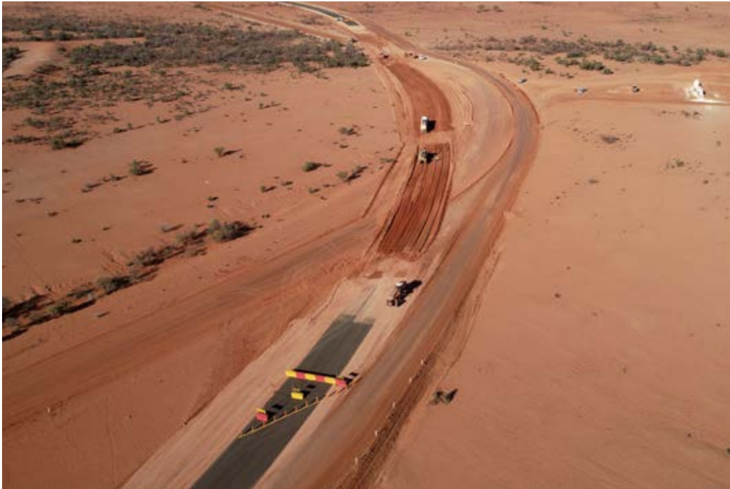
The Silver City Highway being sealed.
