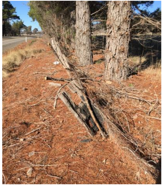
Figure 6-16 View south of fence. Note mortice for rails
