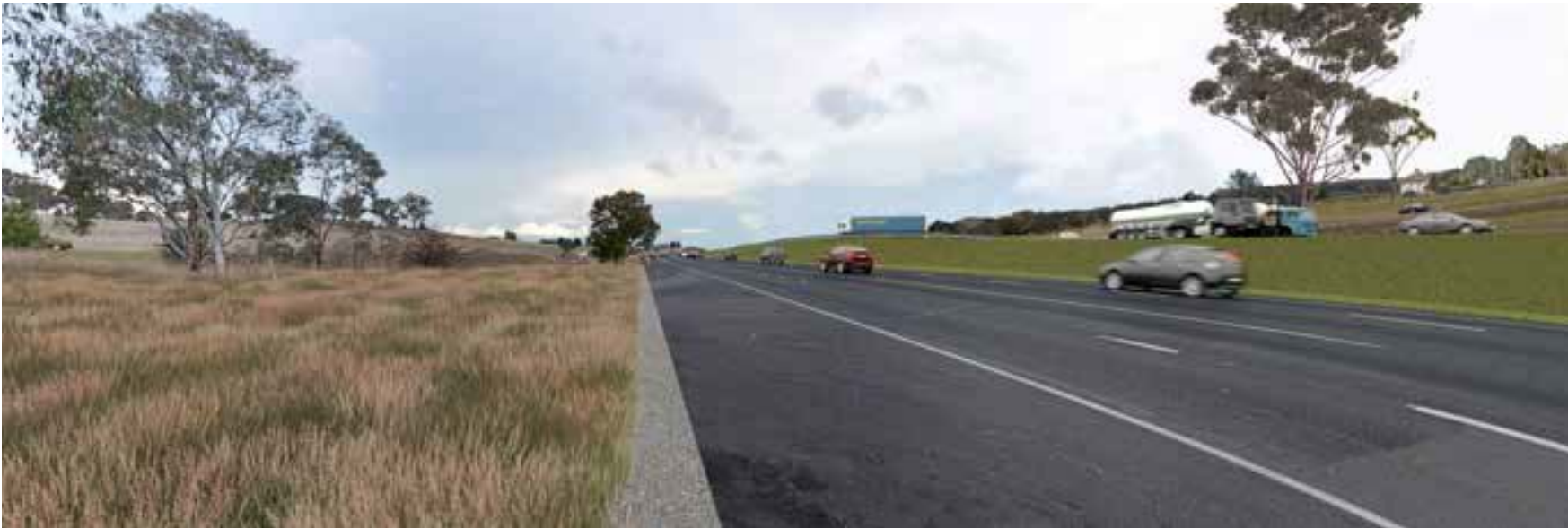
Figure 6-35 Photomontage showing the existing Anchow Hill Lane intersection that would be removed and a new service road provided to the east of the highway
