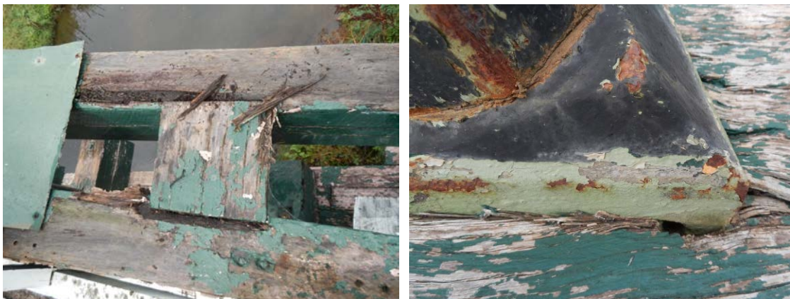
Figure 5-4 Principal rot and crushing (Source: Roads and Maritime)
