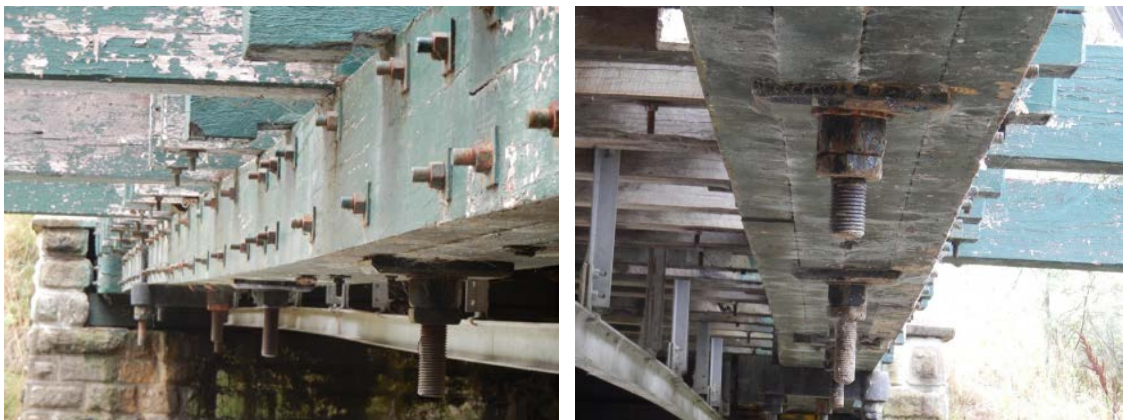
Figure 5-2 Bottom chord loss of alignment (Source: Roads and Maritime)
