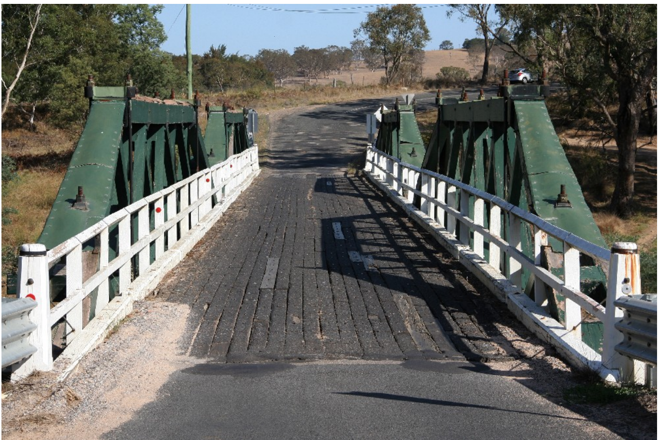
Figure 2-2 McKanes Bridge showing current timber decking
