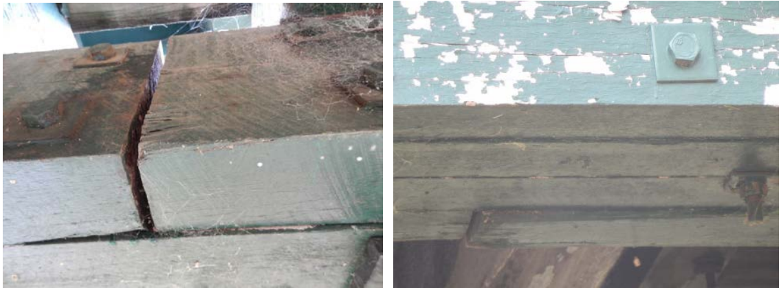
Figure 5-1 Bottom chord flitches opening of joints (Source: Roads and Maritime)
