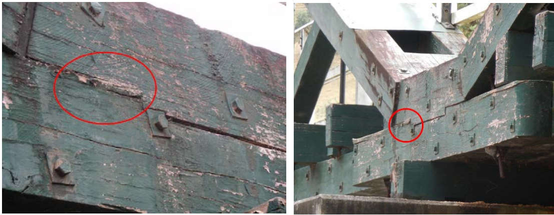
Figure 5-3 Bottom chord shear keys crushing (Source: Roads and Maritime)
