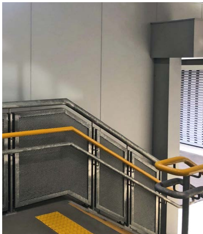
Compliant cladding material was installed at the bottom of the non-fire isolated stairwell
