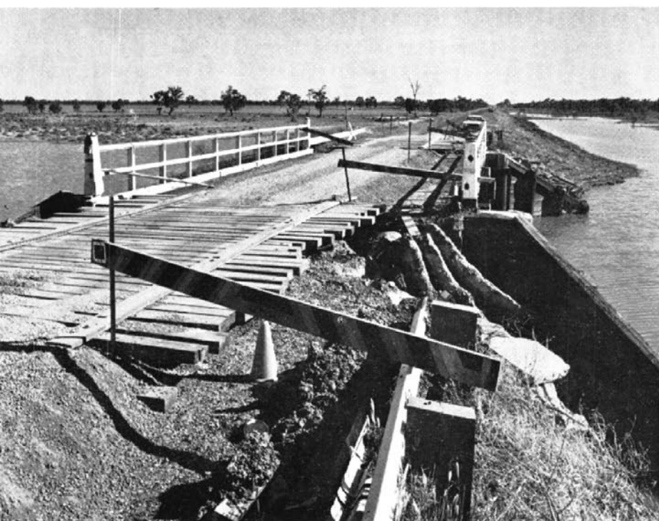
Flood damage to the Castlereagh Highway. Left, just north of Walgett where a box culvert has been washed out. Above, 6.5 km south of Walgett where temporary repairs have been made to sections of road adjoining a bridge. Right, a typical example of eroded pavement, located at 35 km south of Walgett.
