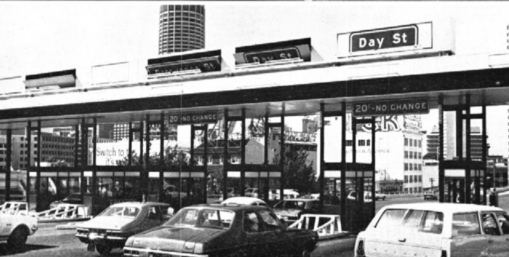
Top left and above: Another movable sign over the southern toll barriers on the Sydney Harbour Bridge is the tilting message board which is raised or lowered to suit the required traffic pattern
