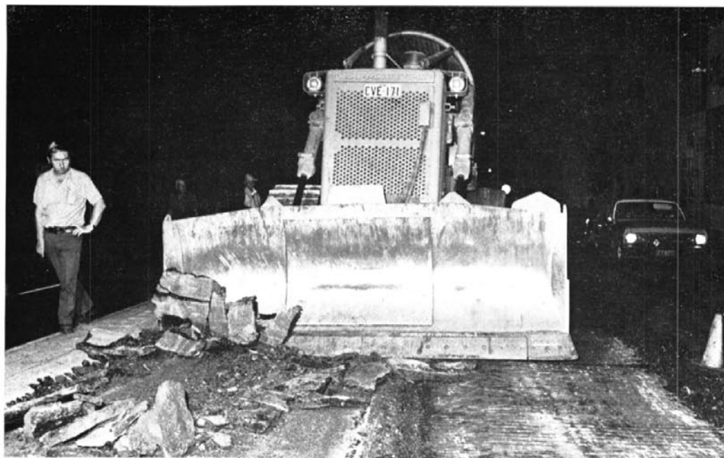
A loader, scraping asphalt against the median strip with a cleared section of carriageway on its left
