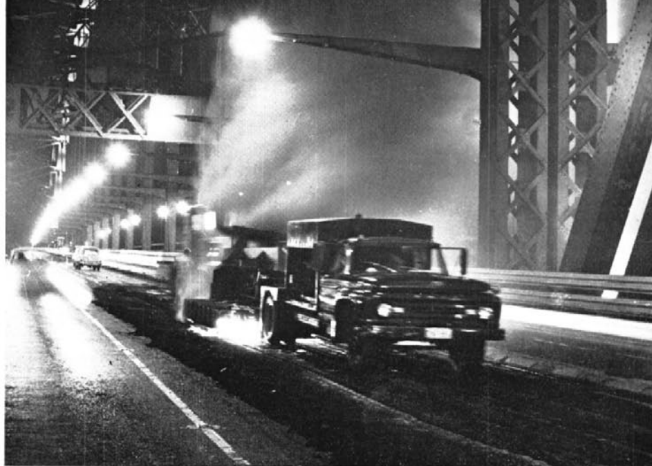
The heater planer at work a few years ago on Sydney Harbour Bridge
