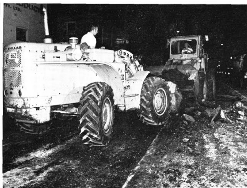
Above: The broadened ripper boot on a Cat D6 Dozer. The sharp pointed toe aids entry into the asphalt for ripping. Right: Two loaders blading loosened asphalt by working towards one another
