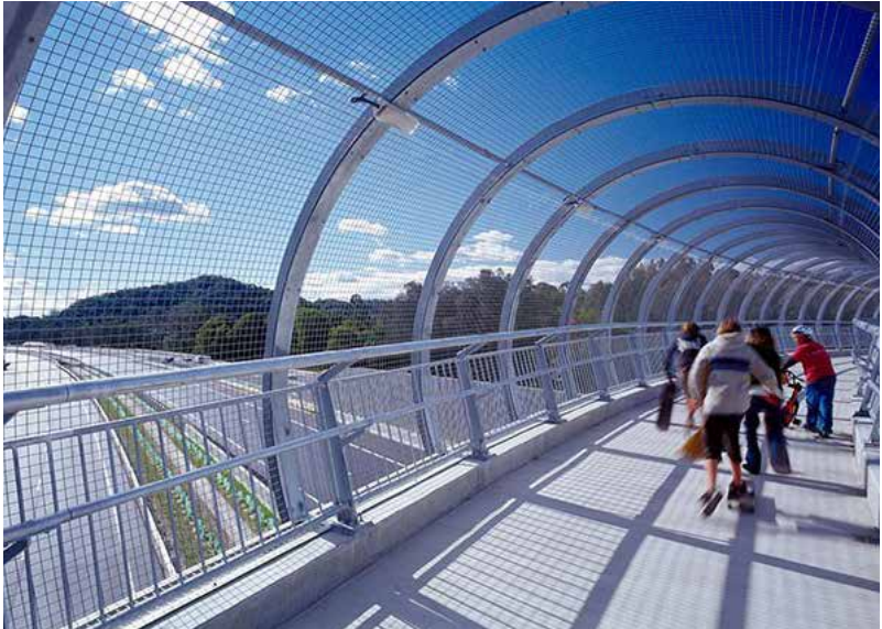
FIG A.10 A FULLY ENCLOSED PEDESTRIAN BRIDGE WITH VISUALLY PERMEABLE MATERIALS.
