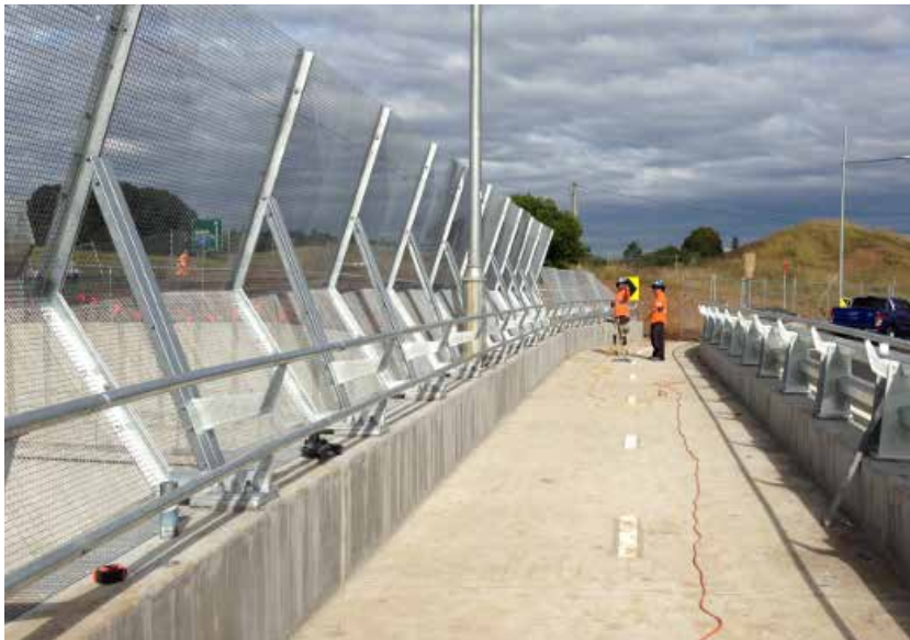
FIG A.8 A THROW SCREEN ADJACENT A BRIDGE WITH PEDESTRIAN FOOT TRAFFIC (BEING INSTALLED).
