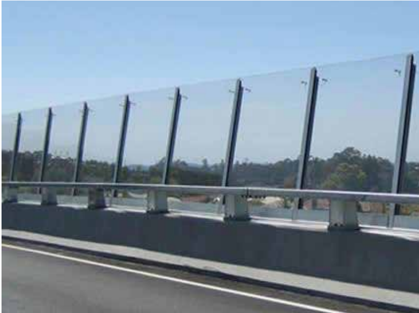
FIG A.5 AN ACRYLIC NOISE BARRIER.
