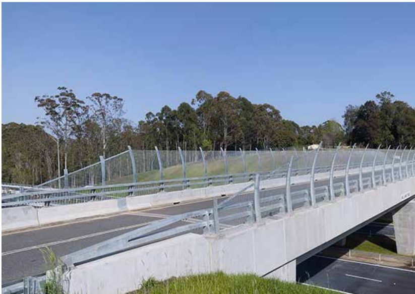
FIG A.7 EXAMPLE OF A THROW SCREEN ON A LOCAL ACCESS BRIDGE.
