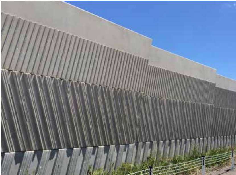
FIG A.6 A CONCRETE NOISE WALL WITH TEXTURE/PATTERNED FINISH.
