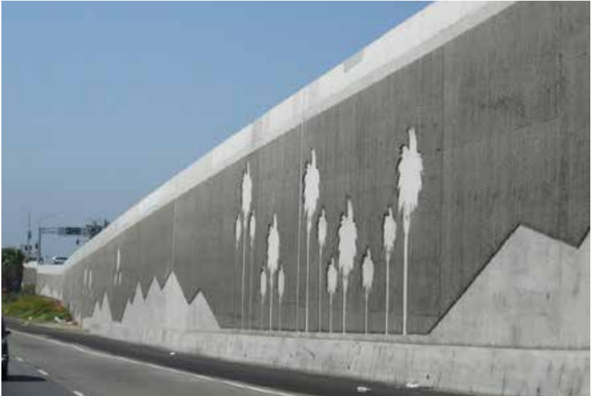
FIG A.9 TEXTURED/PATTERNED FINISH TO A WALL.
