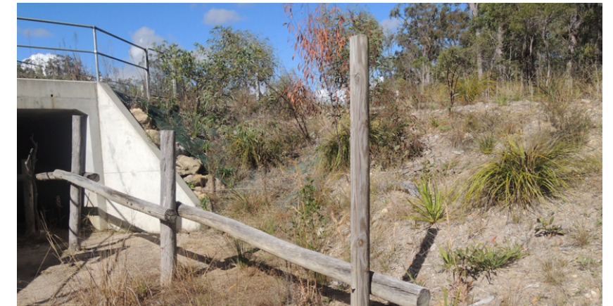
Figure 69: Example of fauna furniture at culvert
