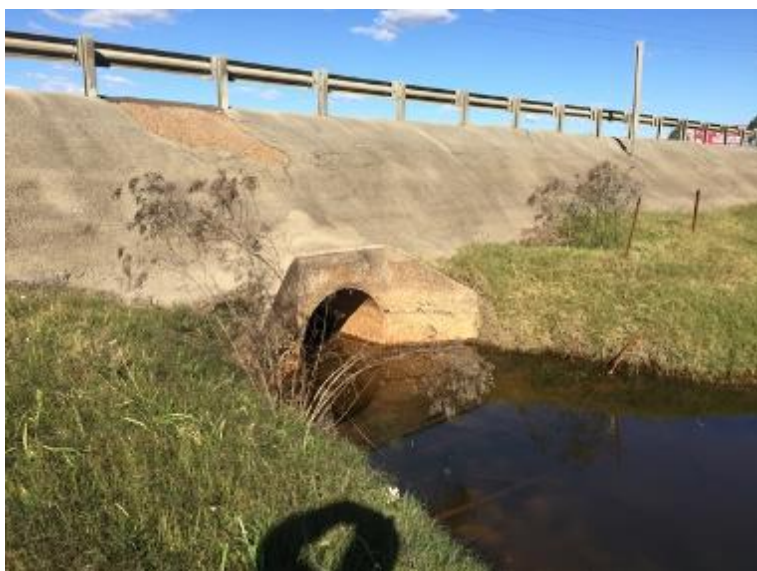
Photo 2-4 Single precast concrete pipe under Cessnock Road
