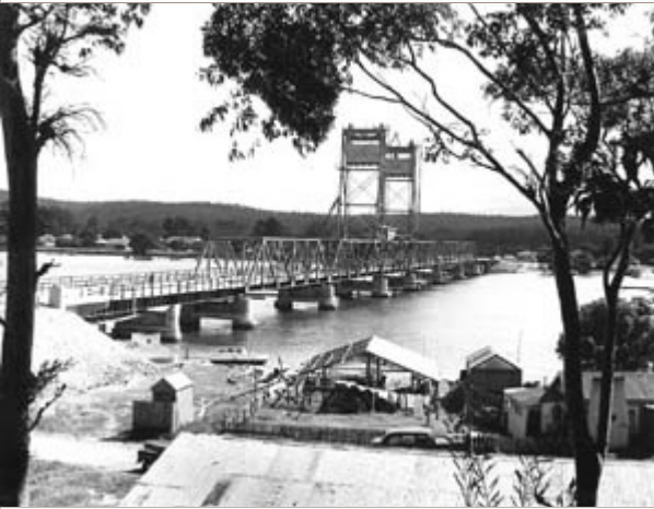
Figure 1-44: Showing the bridge nearing completion. It is constructed with light steel trusses on concrete piers and with a concrete deck. (Nov) 1956
