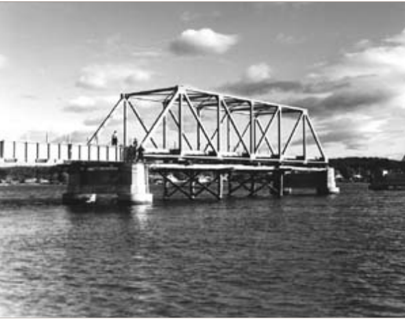
Figure 1-43: First span erected on the bridge over the Clyde River at Batemans Bay (18/8/1955)
