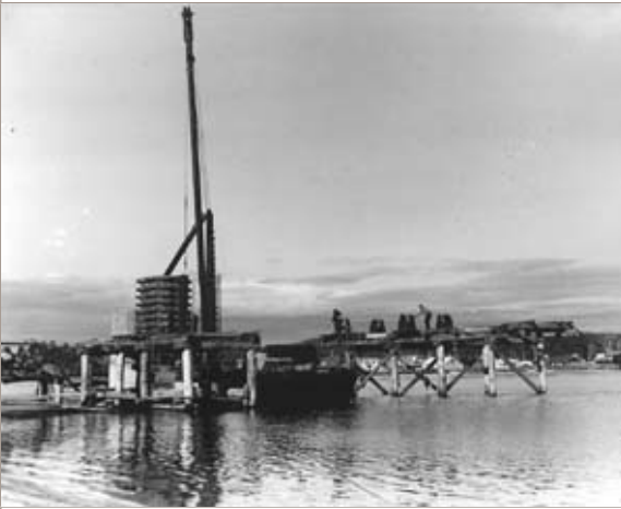
Figure 1-41: Clyde River from northern side looking south toward Batemans Bay. Showing falsework and piers in early stages of construction of new bridge. (26/5/1949)
