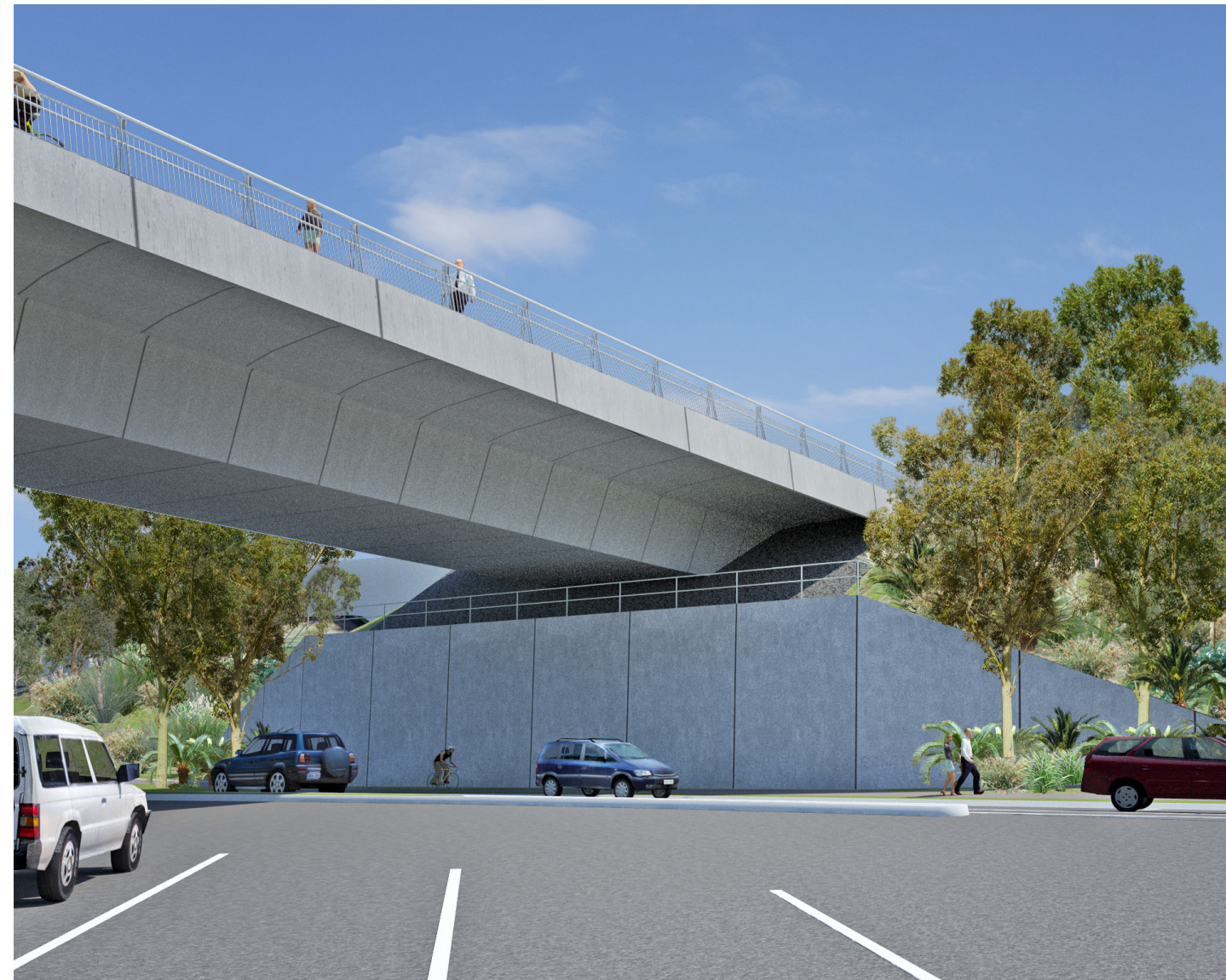
Figure 6-13: View looking towards the northern abutment retaining wall
