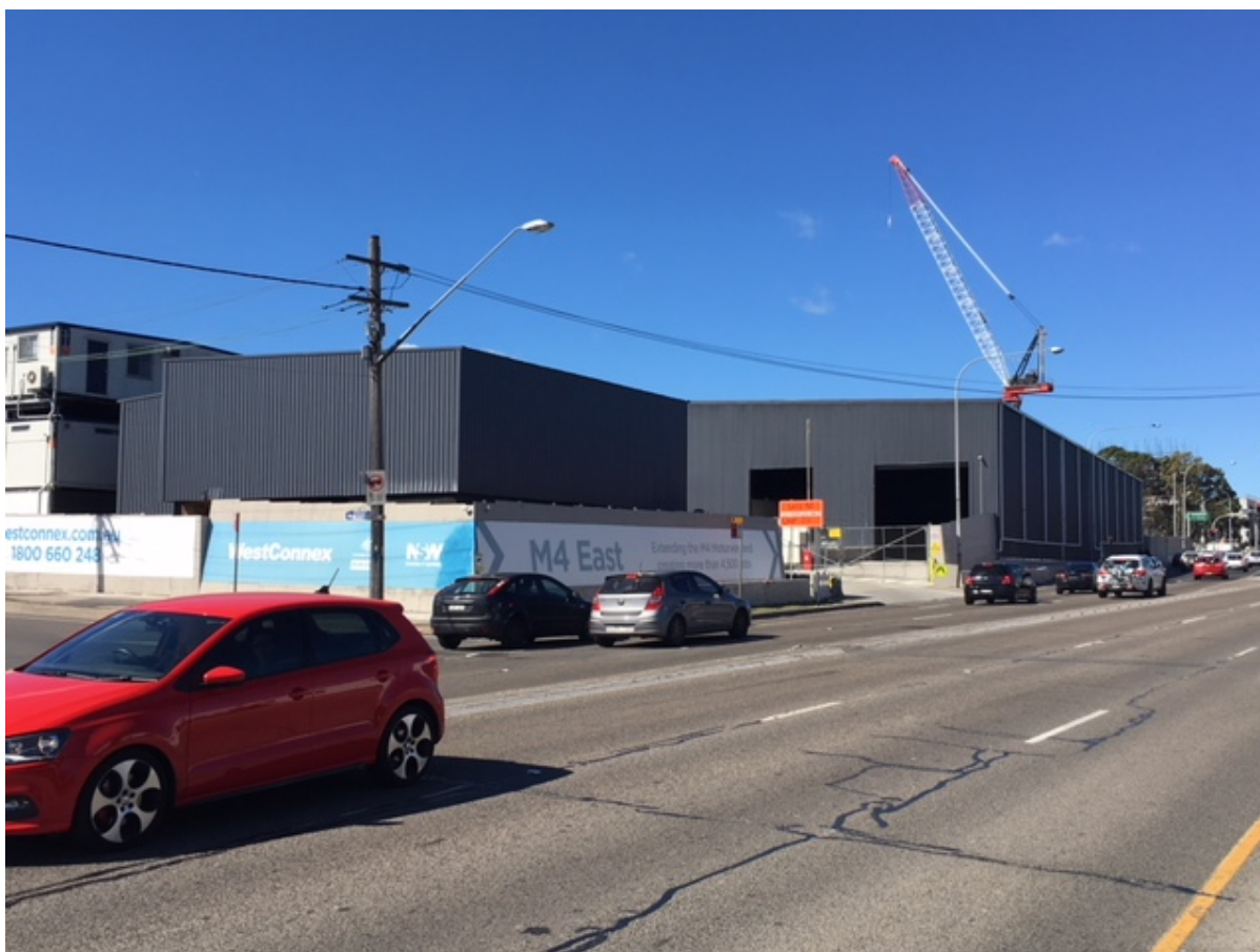
Plate 1 Existing M4 East acoustic shed at the Northcote Street civil and tunnel site
