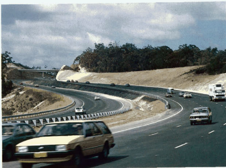
A six lane configuration has been used on the Somersby to Ourimbah section of the F3 — Sydney-Newcastle Freeway because of high traffic volumes and rugged terrain.
