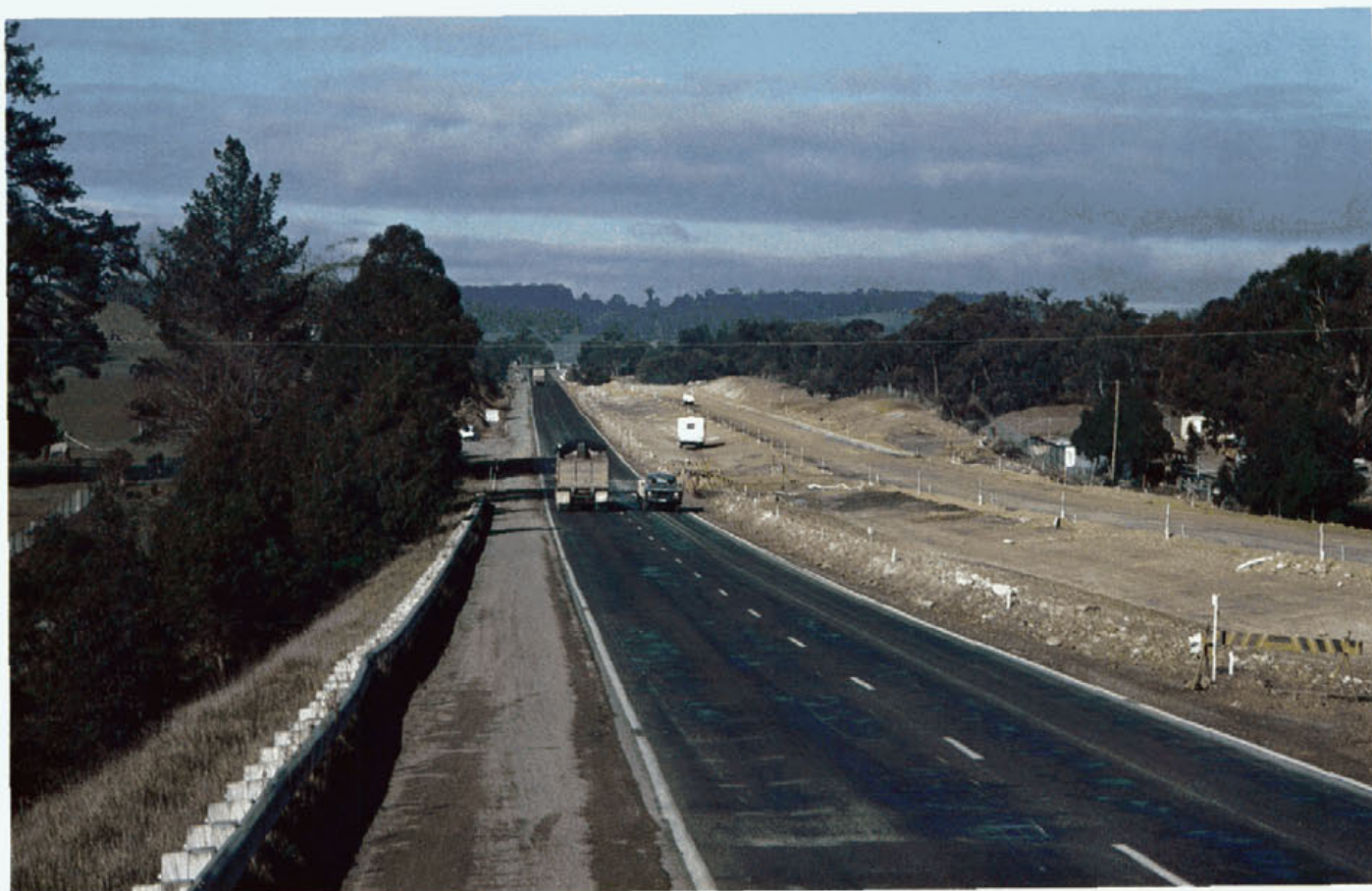
Dual carriageway under construction on the Hume Highway between Black Bobs Creek and Cherry Tree Hill.
