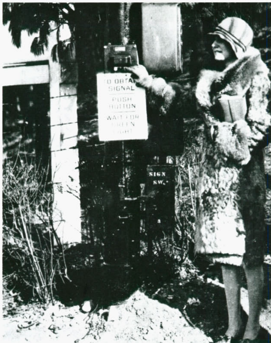
A pedestrian-actuated traffic signal installed in Baltimore, February 1929.
