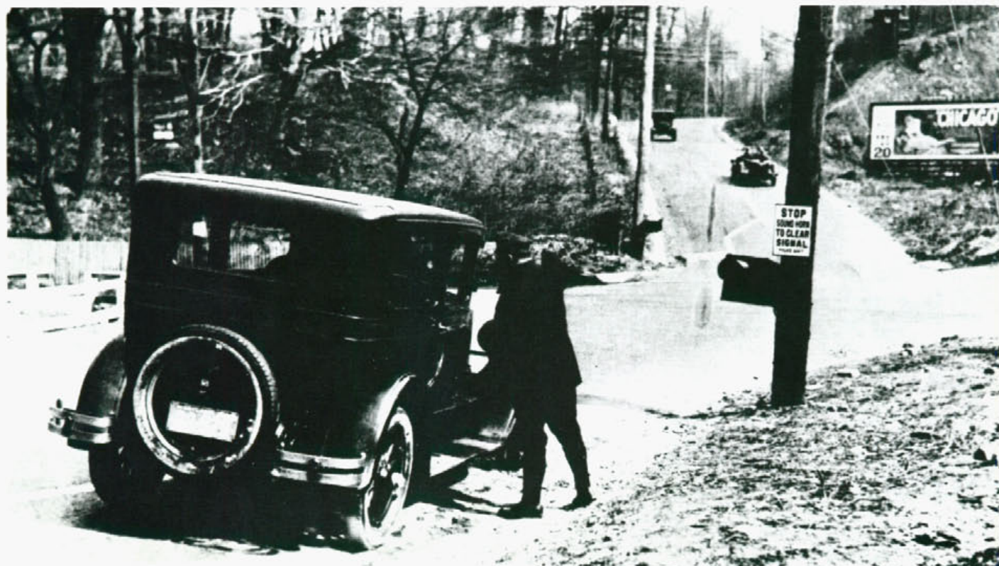
The horn-actuated traffic signal developed by Adler in the U.S.A. in 1928.
