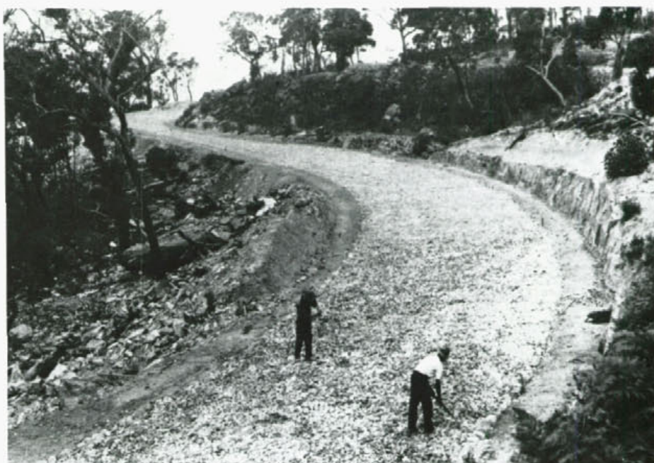
Hand hammers were standard equipment for breaking up the stones on the base course in the 1920s.
