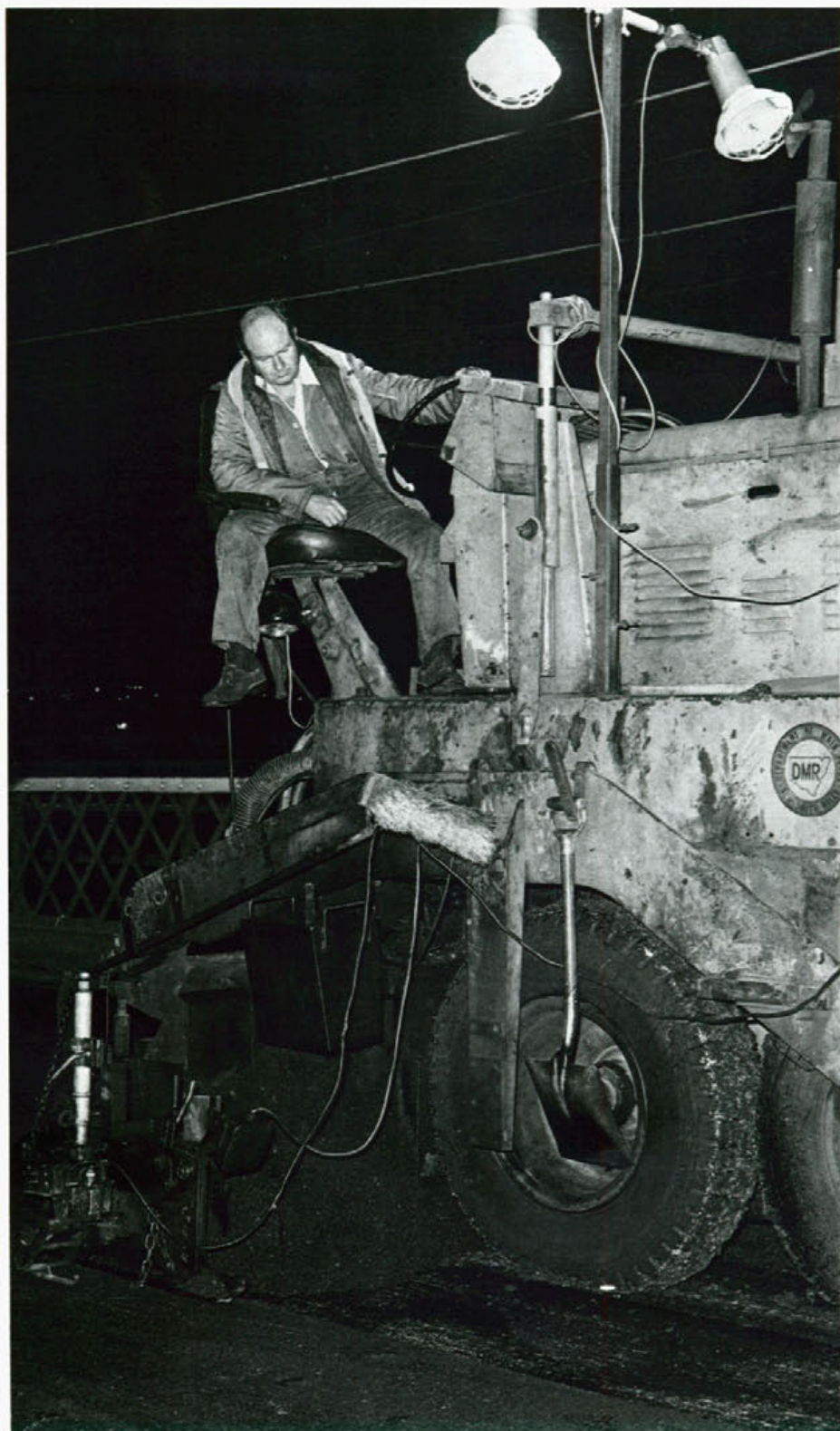
The Department's Rotomill pavement profiling machine cold-milling the old deck surface prior to resurfacing.
