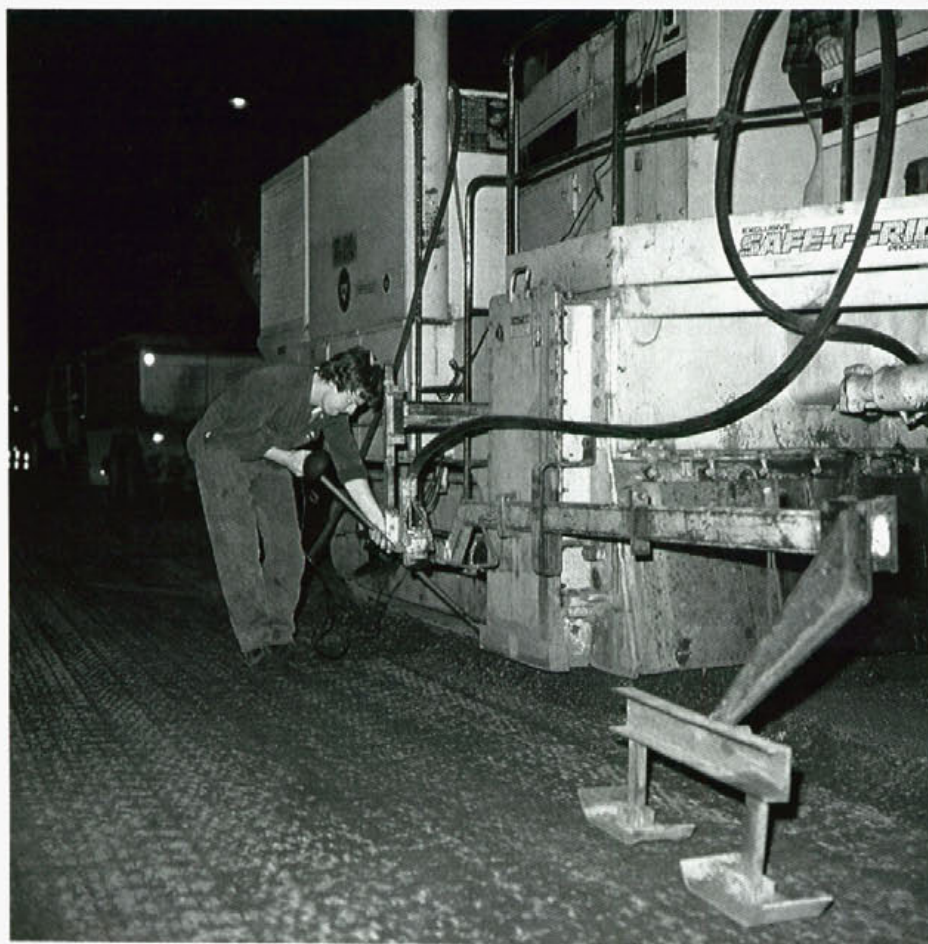
Minor maintenance work being carried out on the Rotomill pavement profiling machine during resurfacing of the Sydney Harbour Bridge. In the foreground is an automatic levelling device.
