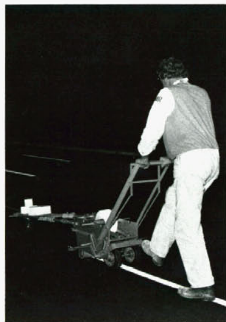
Final touches—hot thermoplastic linemarking material is applied to the new surface.
