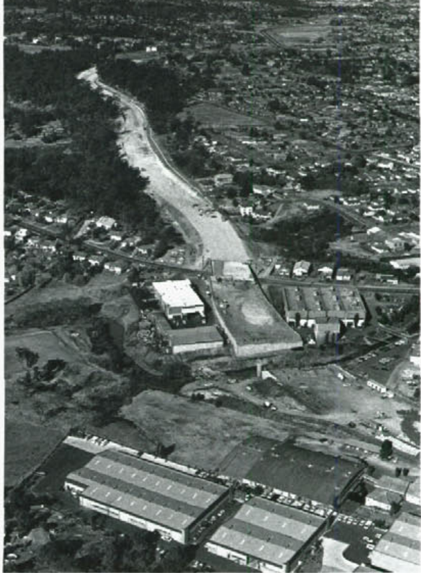
The reinforced earth wall near the North Rocks Road overbridge under construction as at August 1978.
