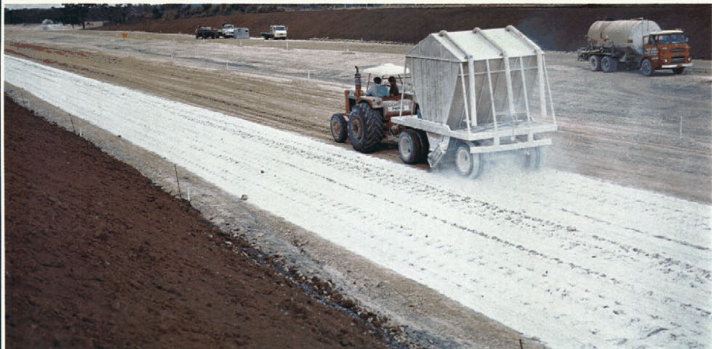
Lime stabilisation on F5. Information on this process and on the equipment used is presented in the preceding article.
