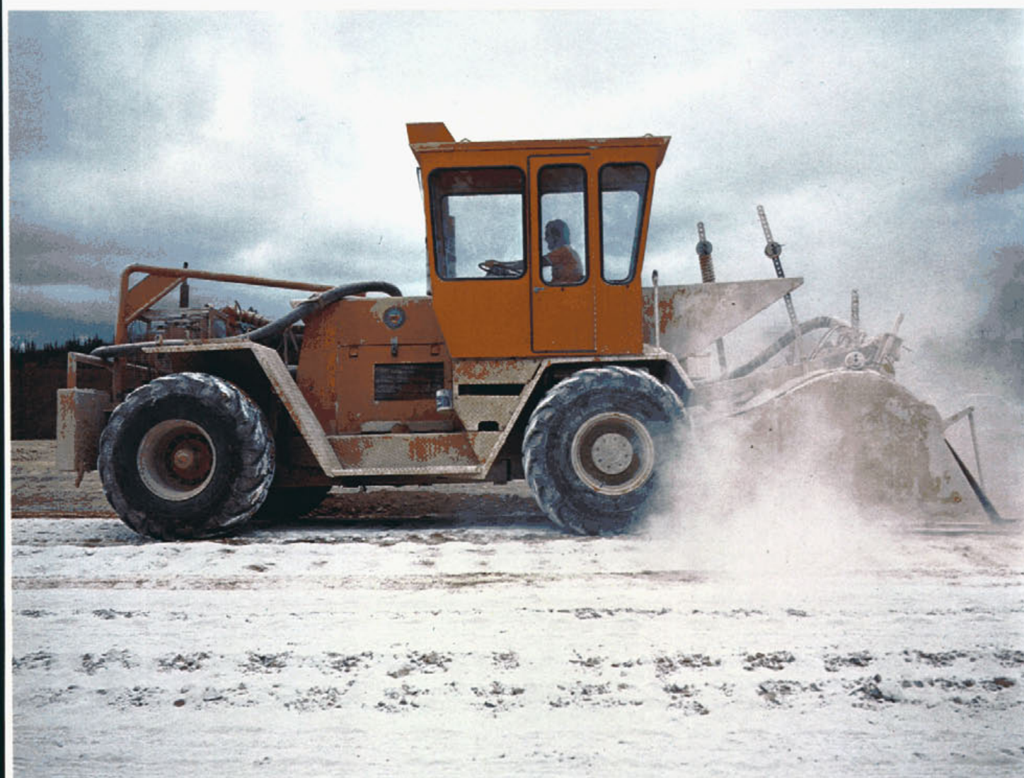
Lime stabilisation on F5. Information on this process and on the equipment used is presented in the preceding article.
