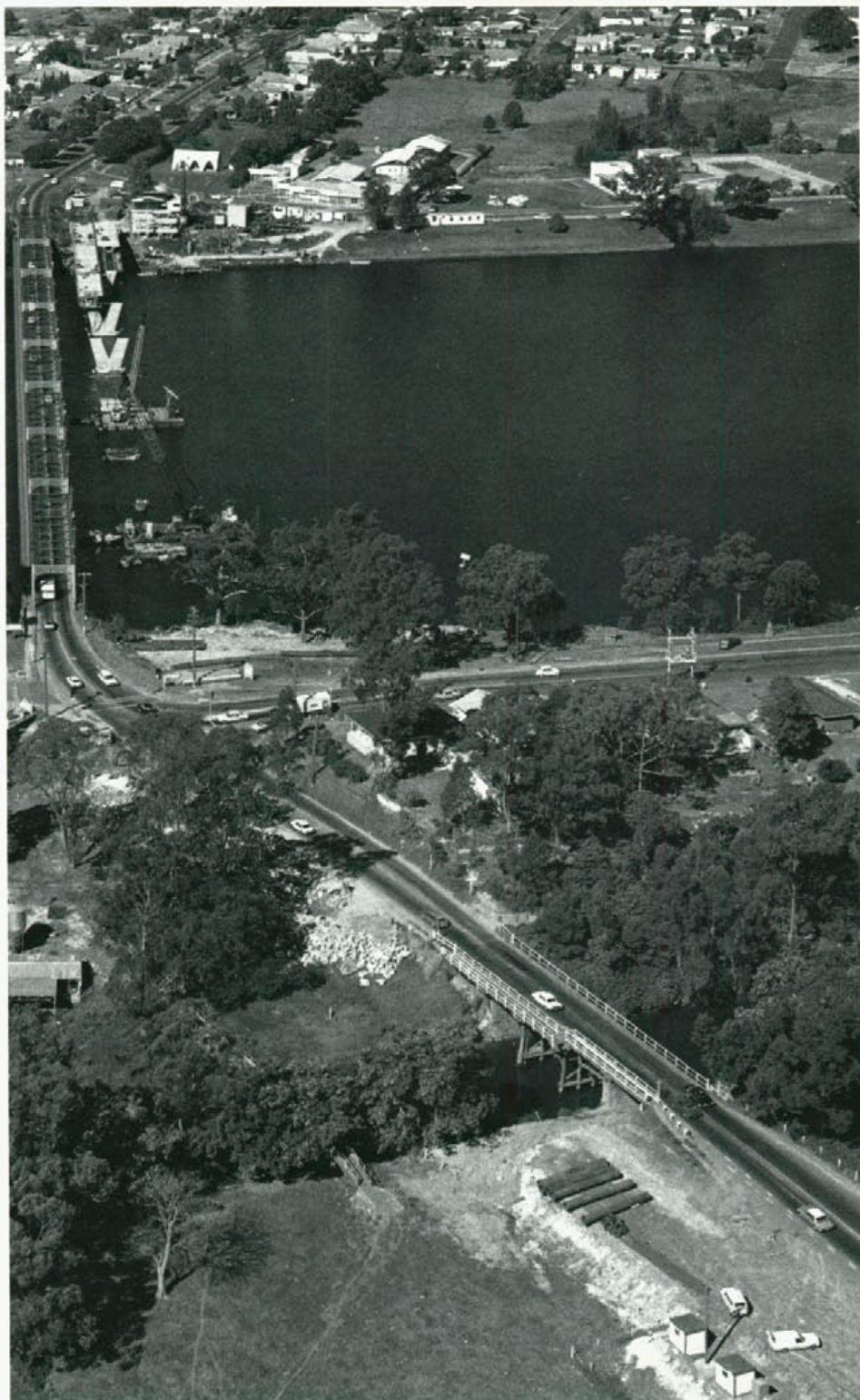
Construction of the approaches to the bridge over Bomaderry Creek as at April 1979. The new bridge being built over the Shoalhaven River can be seen in the background.
