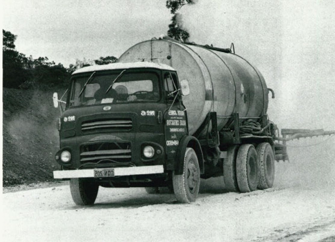
A water tanker hydrating lime on a section of the F5 — South Western Freeway
