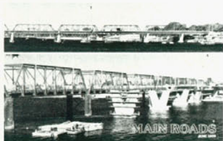
Cover: Two views of the new bridge over the Shoalhaven River at Nowra, being built alongside the existing 1881 structure. (See feature article on pp.98-106).
