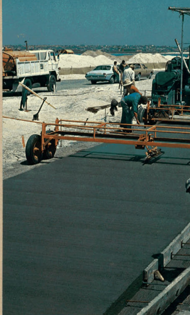
The Stothert and Pitt CPP 60 slip-form paver at work on 140 m 3 /day (8 hours). Pavement texture for maximum to the second trailer. The first trailer held a platform for
