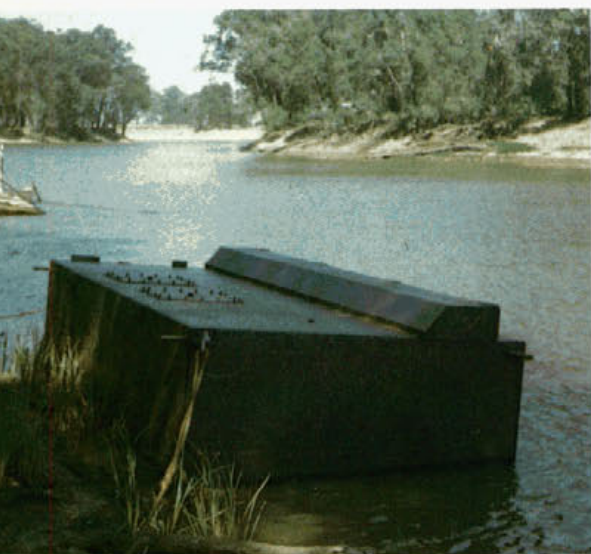
The first steel pontoon lies in the river awaiting assembly.
