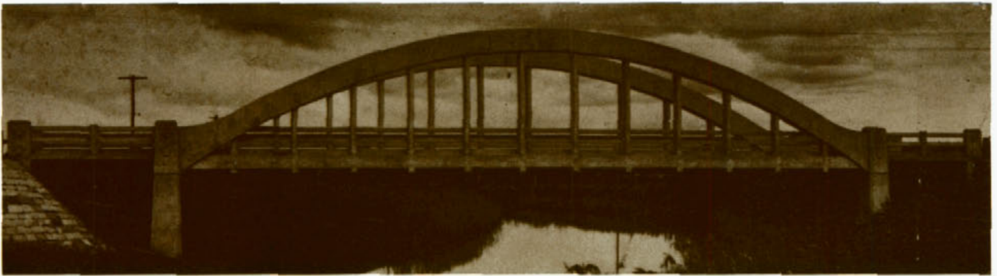
This reinforced concrete bowstring arch bridge over Shark Creek on the Pacific Highway near Maclean was completed in 1936 and was the first of its type to be built in New South Wales. The design by the Department was also noteworthy, being the first to introduce temporary hinges in the arch rib to avoid moments from rib compression and extension of the tie. An article on this bridge appeared in the May 1936 issue of "Main Roads", Vol. 7, No. 3, pp. 89-91.
