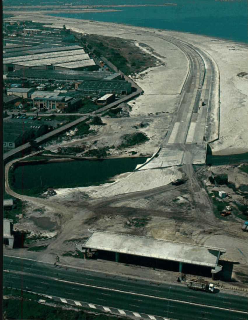
Construction at the north-western end of The Foreshore Road near its junction with General Holmes Drive. The elevated decking in the foreground will eventually carry General Holmes Drive's southbound carriageway over The Foreshore Road.
