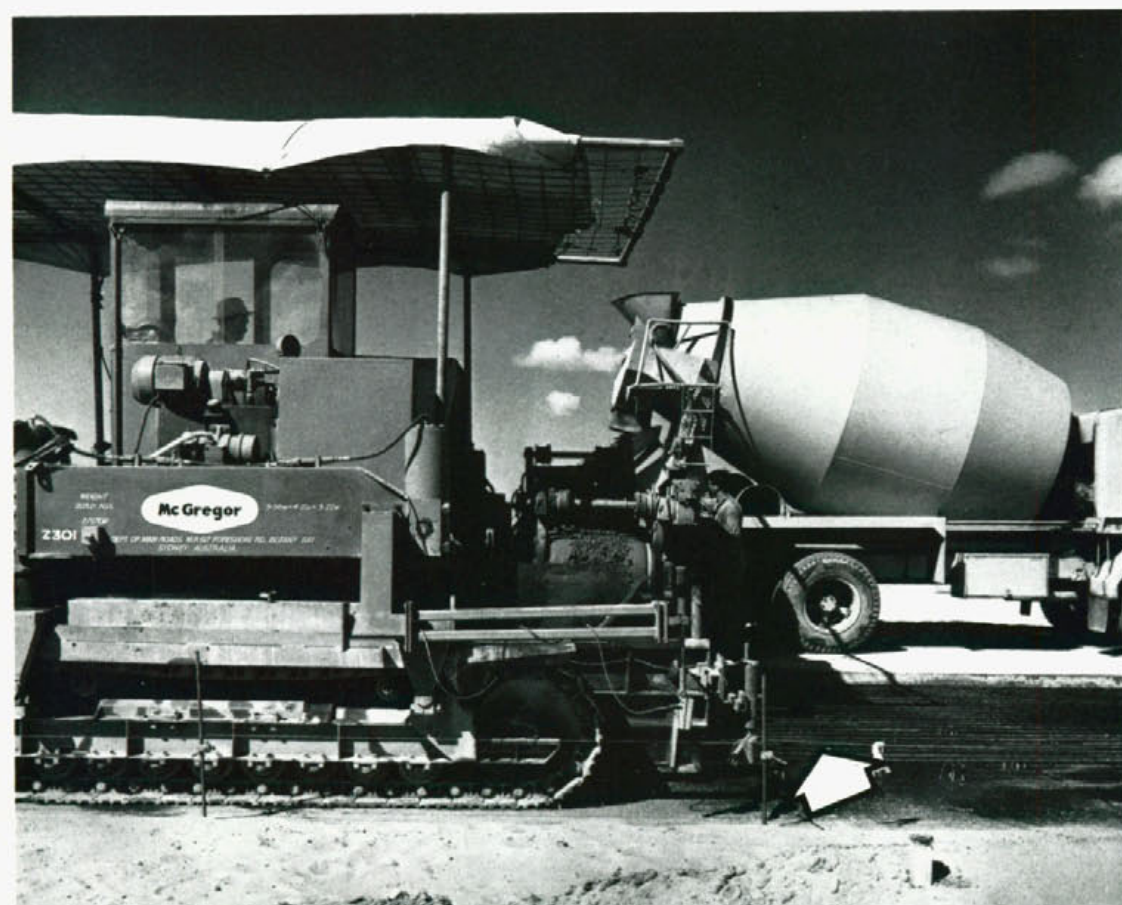
A constant supply of concrete was necessary to maintain uniform pavement qualities. The taut stringline (arrowed) was used to guide the paver.
