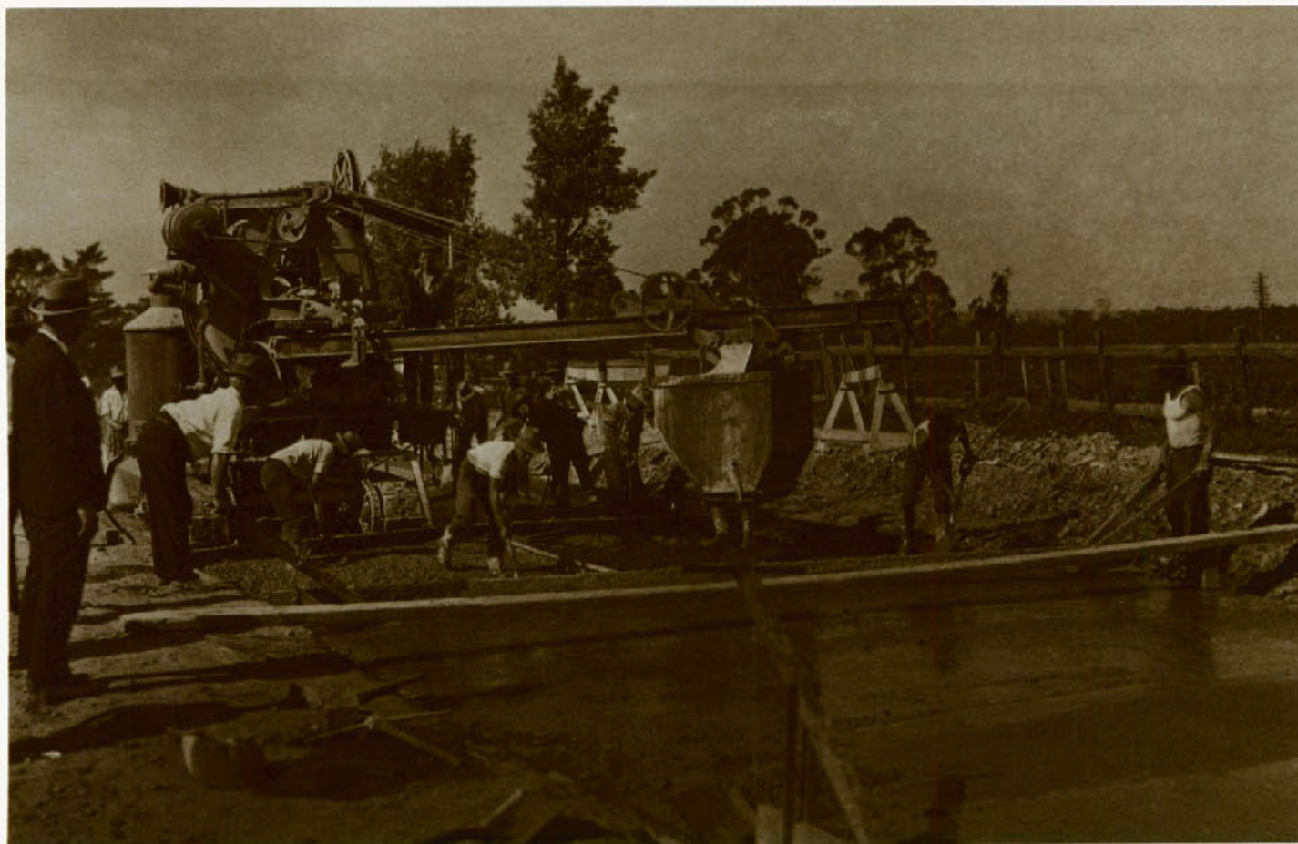
Once poured, the concrete is spread and finished by hand.
