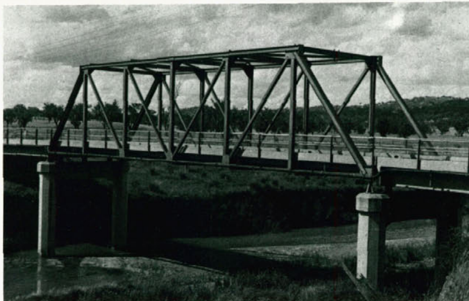
The only all-welded steel truss span built by the Department was for this bridge over the Manilla River at Barraba on the Tamworth-Barraba Road, completed in 1935. An article on the bridge and the comparison of designs for riveted and welded truss spans appeared in the May 1936 issue of "Main Roads", Vol. 7, No. 3, pp. 111-114.
