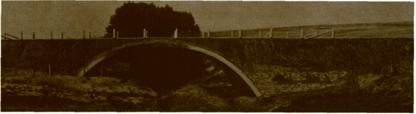
At the time of its construction in 1930, this bridge over Walkers Creek, on the Barton Highway, was the largest reinforced splayed arch road bridge in Australia. An article describing its construction appeared in the October 1931 issue of "Main Roads", Vol. 3, No. 2, pp. 28-9.
