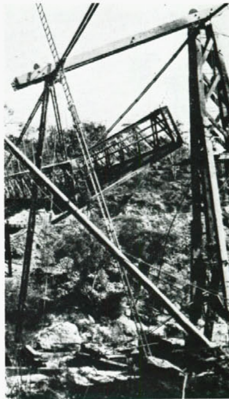
Another view of the damaged bridge showing the suspended span and the damaged upstream tower at the Maldon end. The downstream tower was completely destroyed, as was the timber deck and three approach spans.
