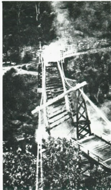
A view of the suspension bridge from the Maldon end immediately after the fire in January 1939, showing portions of the structure still smouldering.
