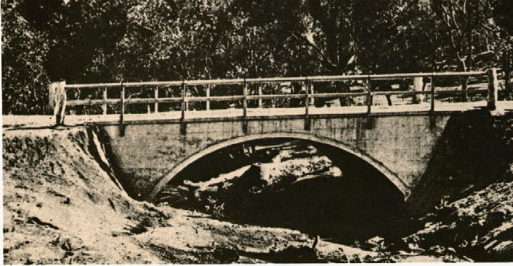
"Monier" Arch Bridge over Read's Gully on the Main Northern Road near Tamworth in 1900. Reproduced from the Journal and Abstract of Proceedings of the Sydney University Engineering Society for 1900, Vol. 9, page 65 by courtesy of the Fisher Library, University of Sydney.
