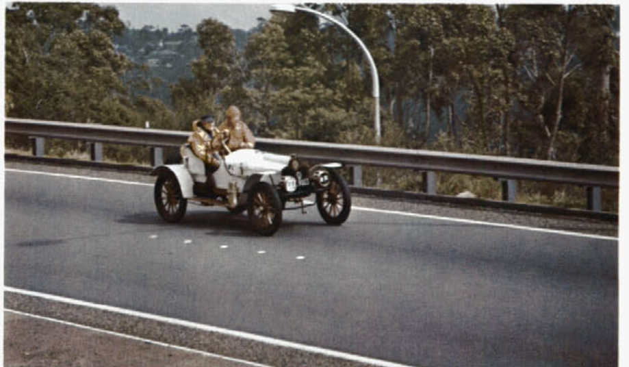
Below: The seven decades, which have passed since the era of this Sizaire Naudin, have produced such new features as electric street lighting, safety fencing, divided carriageways, raised medians, improved road base construction and surfacing, "rumble" strips and breakdown lanes, reflectorised and raised lane markings and many more.
