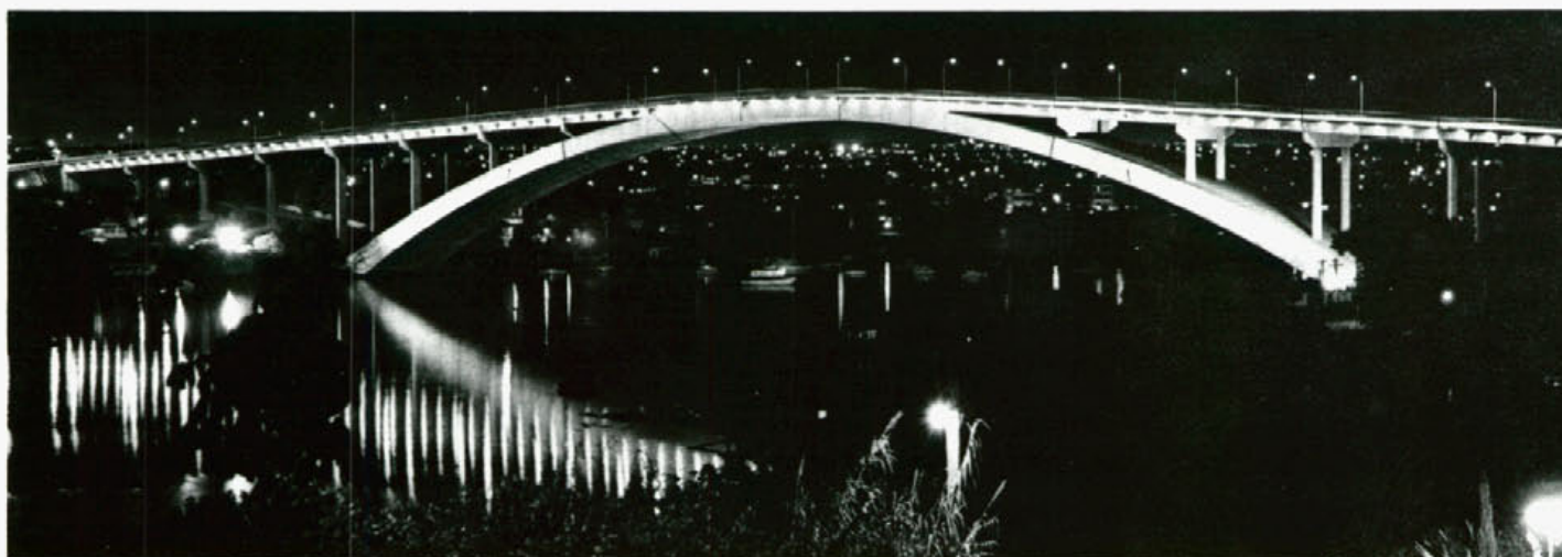
Above: Gladesville Bridge is another record-holder — being the world's longest concrete arch span with a leap of 305 m. The bridge was opened on 2 October 1964 and is shown here specially floodlit for the opening of the Sydney Opera House in 1973.
