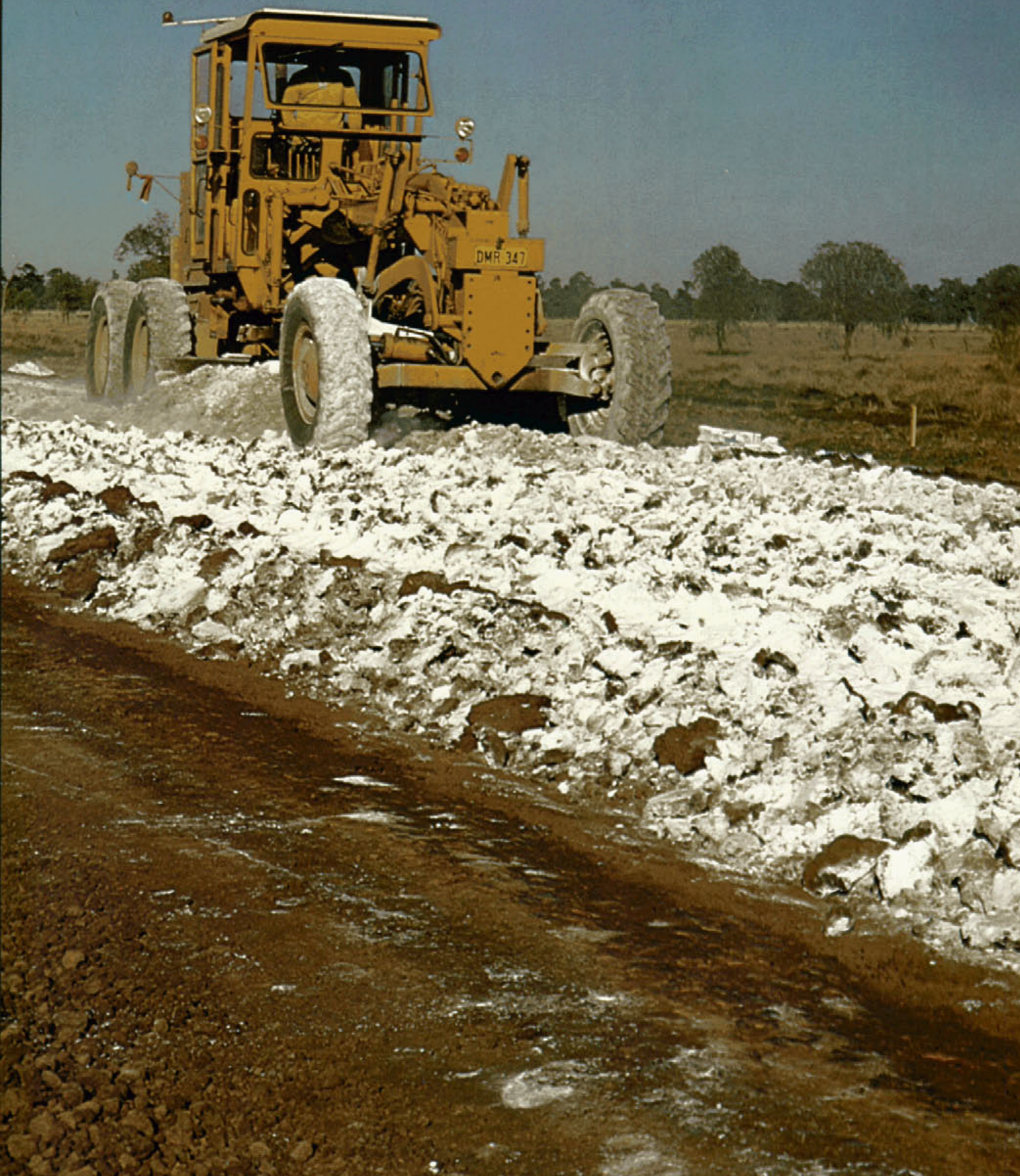
A grader mixing lime into gravel to form a stabilised road surface on the Newell Highway between Moree and Boggabilla.
