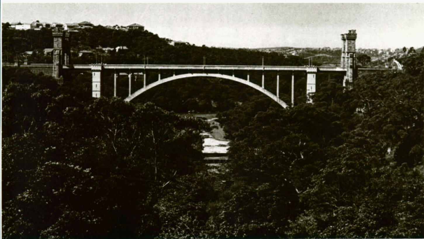
The size of the reinforced concrete arch span beneath the deck of Northbridge "Suspension" Bridge can be appreciated from this photograph. The original bridge was built by a private company about 1892. When the Department found the suspension cables to be corroded, it converted the bridge to an arch structure in 1937-39.
