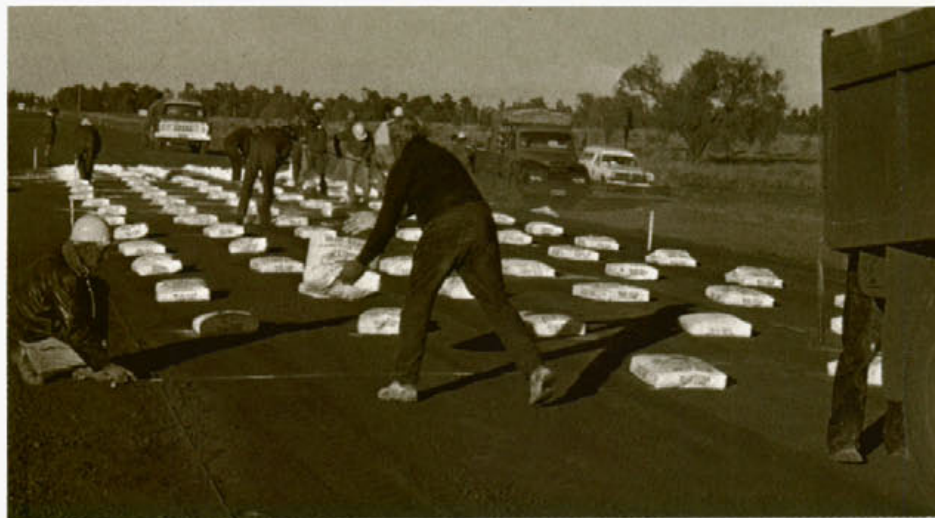
Above: Placing bags of lime in position on the gravel pavement prior to spreading.
