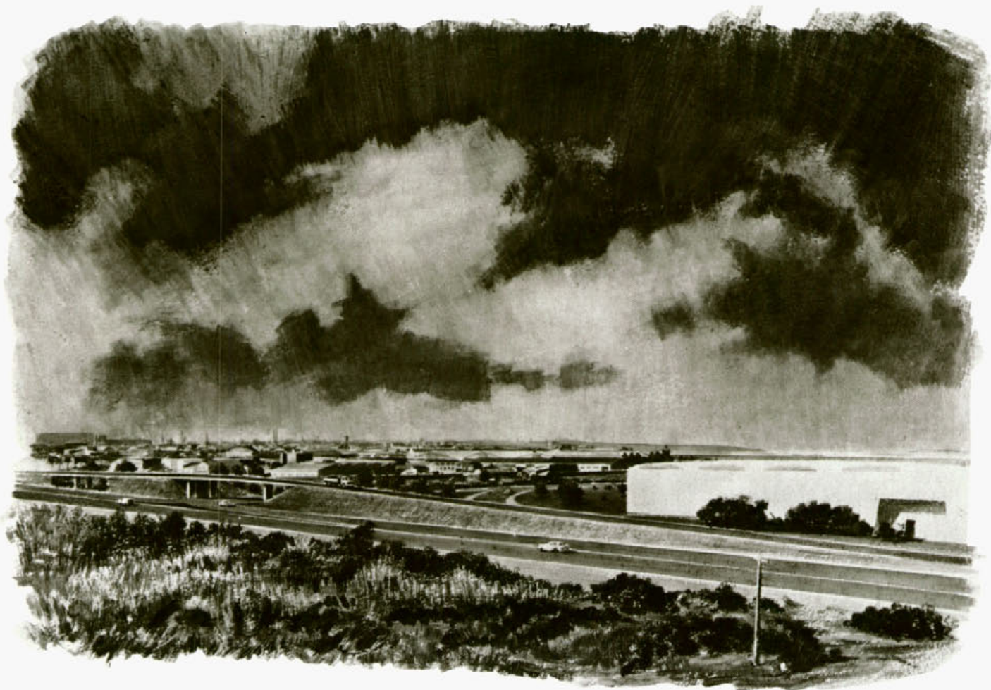
An artist's impression of the junction of the new Foreshore Road and General Holmes Drive. It shows the bridge which will carry the southbound carriageway of General Holmes Drive over the access links between the northbound carriageway and the Foreshore Road. The building on the right is the Maritime Services Board laboratory.
