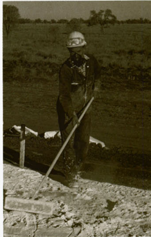
Above: Placing bags of lime in position on the gravel pavement prior to spreading.
