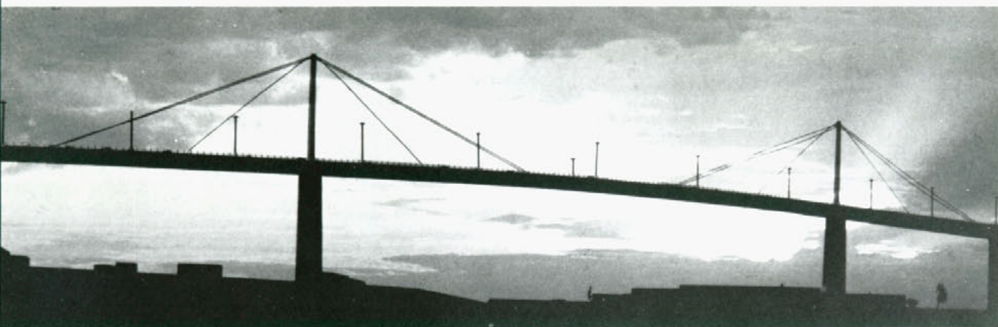
Above: An artist's impression of the central portion of Melbourne's new 2583 m long West Gate Bridge, which is due to be opened late this year, and is already a dominant feature of the skyline at the mouth of the Yarra River. This will be Australia's second road bridge with a cable-stayed span, and will also be the country's second longest single span.
