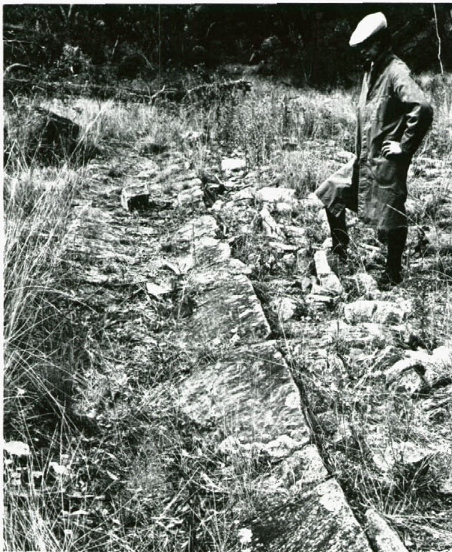
Overgrown with grass and moss, this section of a basalt slab table drain bears testimony to the workmanship of early road builders.
