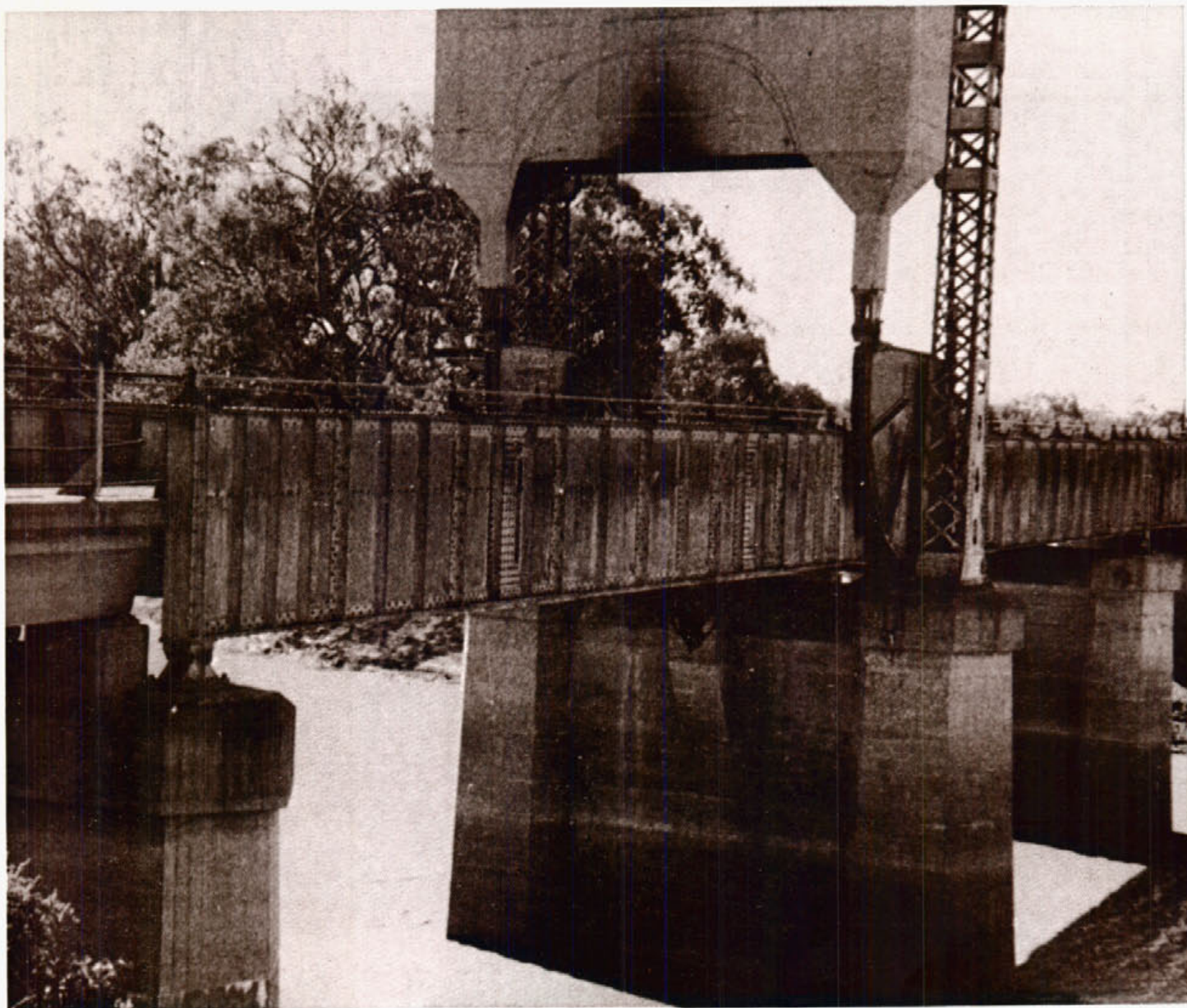
Taken in 1958, this photograph shows the concrete counterweight and the associated towers. At this time the lift span had been immobile for 11 years. The counterweight and towers were removed in 1970 to give sufficient clearance for trains carrying semi-trailers between Parkes and Western Australia.
