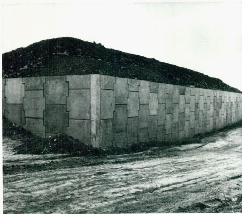
This reinforced earth retaining wall at Menangle, was the first of its kind to be completed by the Department. The wall is part of the abutment works for the bridge carrying the F5—South Western Freeway—over the Main Southern Railway Line at Menangle, about 56 km south of Sydney.
