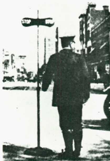
This early "manipulating semaphore" in Detroit was clearly one of the simplest of mechanical signals and one of the early moves away from traditional arm and hand movements.
