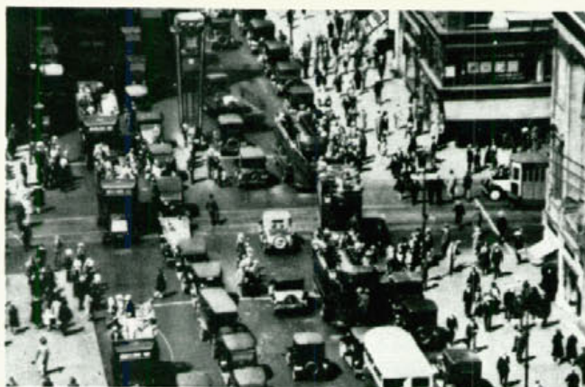
Left: This type of tall traffic tower was in vogue in the United States in the 1920's. This one in Detroit used twelve 250 watt lamps to illuminate the top red, amber and green signals, and eight 96 watt lamps in the lower "driver-eye-level" lights which showed red and green only.
