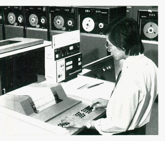
The installation of the second of the Series 2000 machine, a H.2040A central processor (replacing the H.1200 machine) was made early in August, 1975. Eight Model 277 disk drives (64 million character capacity) were placed on site at the same time but will not come into operation until a new air-conditioning system has been commissioned early in 1976.
