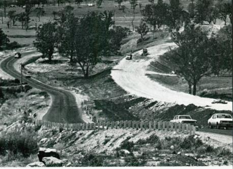
(Above): Reconstruction on the New England Highway, 3.5 km south of Muswellbrook, where this winding section will be eliminated on completion of a new section on an improved alignment and grading.
