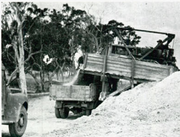
Before the development of front end loaders two methods of loading were the chinaman loading ramp and the side loading ramp.
