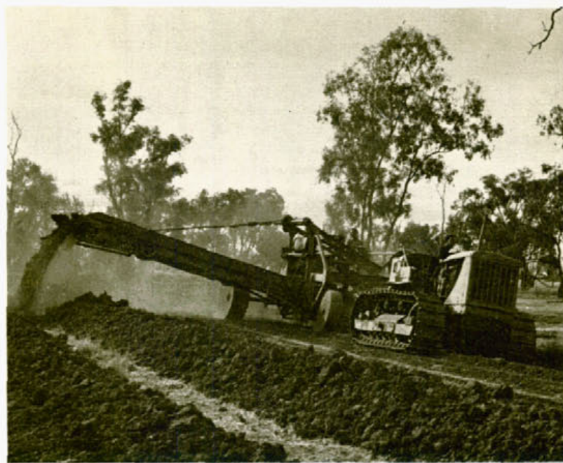
A 6-cylinder, 54 kW, diesel-engined elevating scraper drawn by a 70 kW tractor constructing an elevated formation in 1954.
