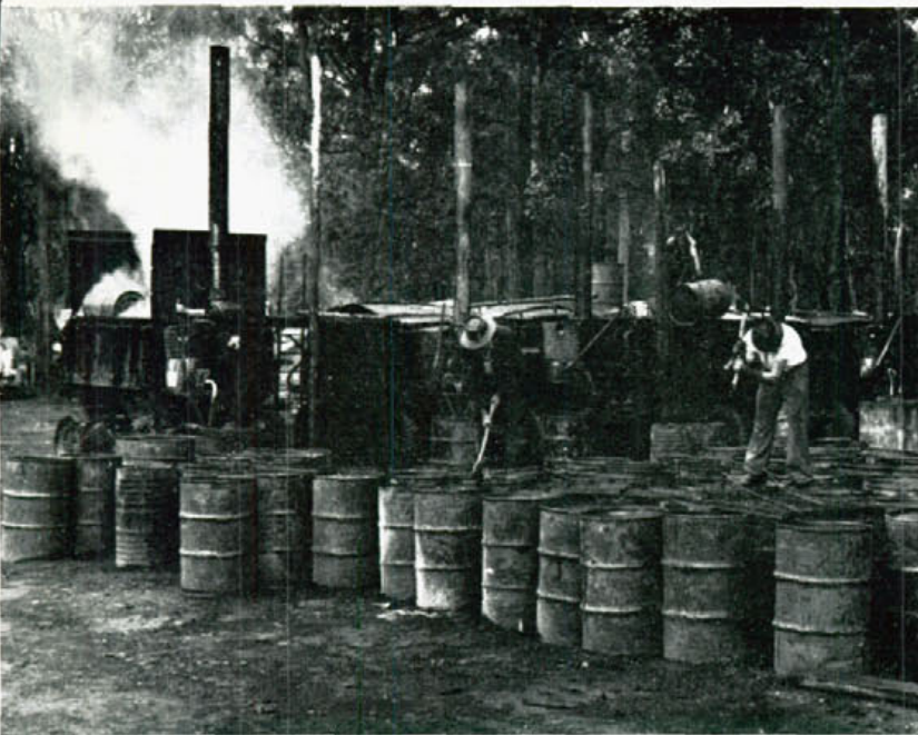
In this 1947 photograph, six kettles heat bitumen ready for use on the roads.
