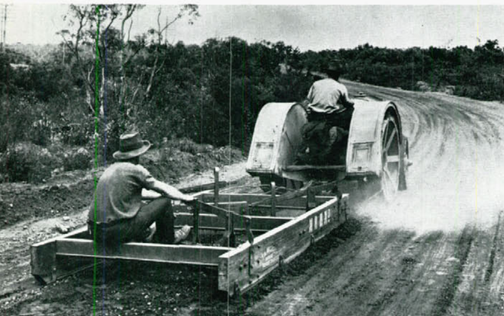
A 1927 method of grading using a planer drag compared with the modern dual lane automatic trimmer spreader, seen here involved in a trimming operation.
