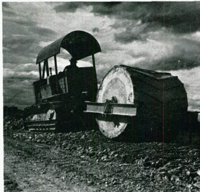
Breaking up shale with a cleated roller which is being pulled by a 40 kW tractor. This photograph was taken in 1948.
