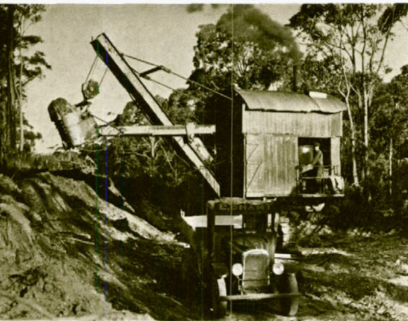
A steam shovel of about 0.75 cubic metres capacity operating in 1938.
