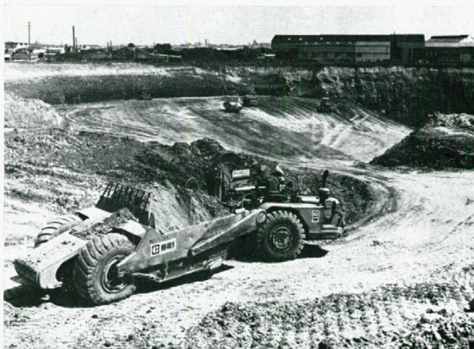
Portion of the "Brick Pit", on the eastern approaches to Duck River Bridge, is being filled to the natural surface level.
