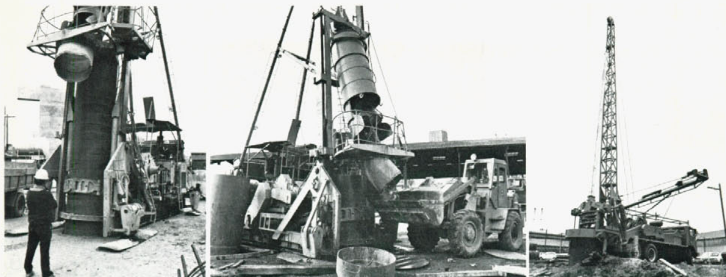
Above: A semi-rotary alternate movement drives the tube downwards. The interlocking tubes come in lengths of 6 m but their width varies
