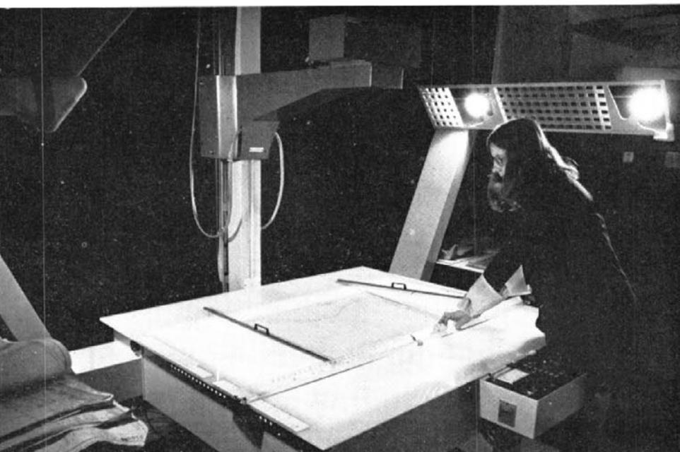
The versatility of the Planetary Camera makes it ideal for the variety of older drawings of differing quality.
