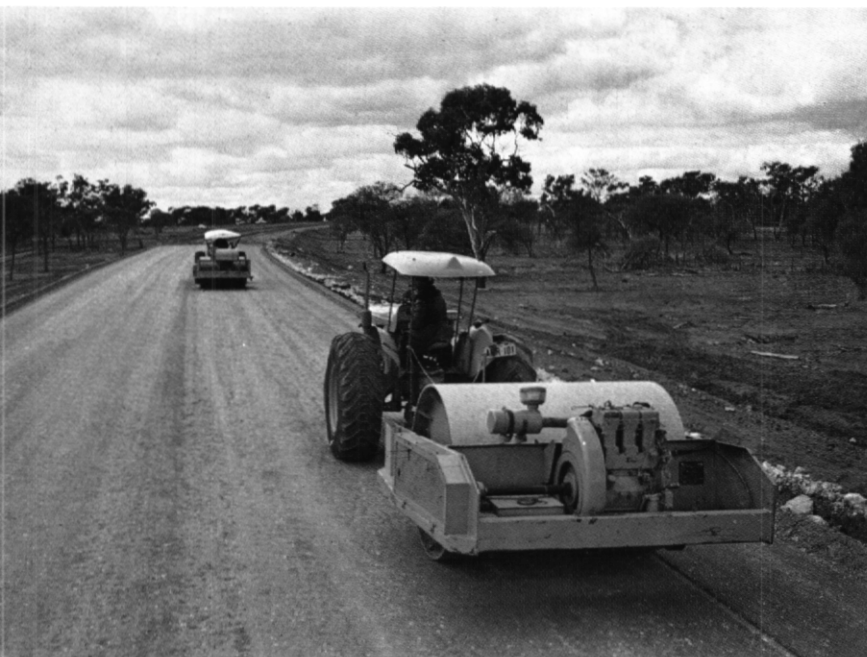
Vibrating rollers compact Maccullochs Range deviation during construction
