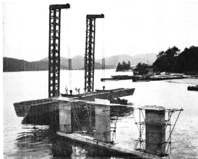
Hawkesbury River Bridge First girder being placed in position
