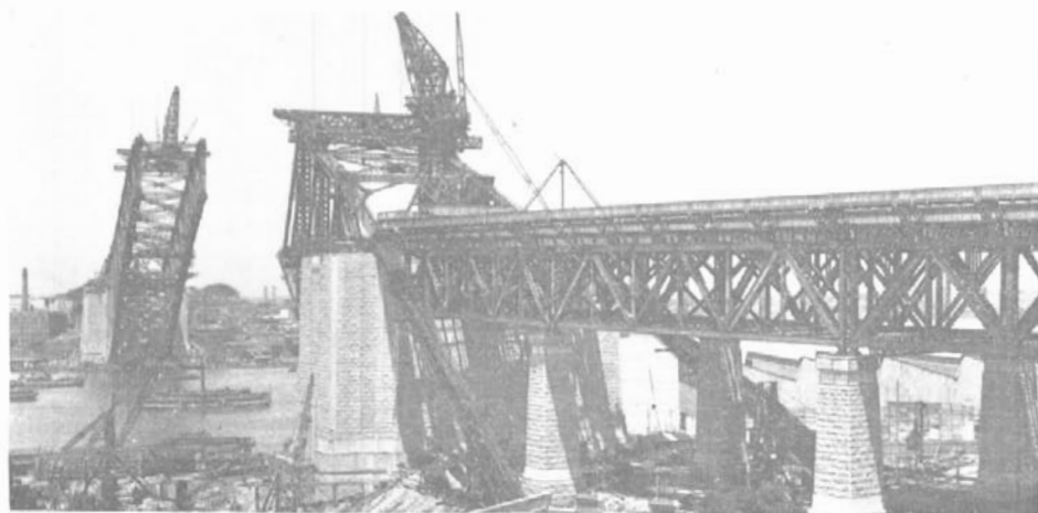
View from northeast showing northern approach spans, creeper cranes and cables which anchored each half-arch during construction. 2nd January, 1930
