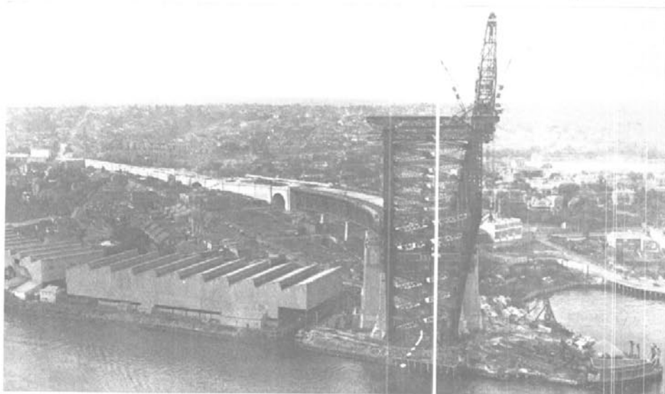
View from southern half-arch, showing nine panels in place on north side. The fabricating shops (often referred to as "Dorman's tin sheds") can be seen on left. 1st April, 1930
