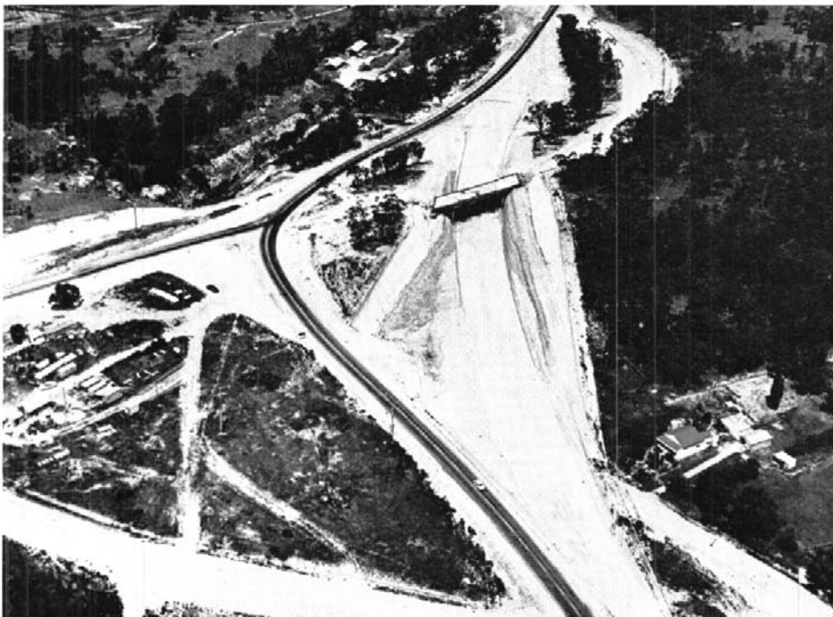
Closer view showing construction of the overbridge to carry Mudgee-bound traffic over the Great Western Highway.
