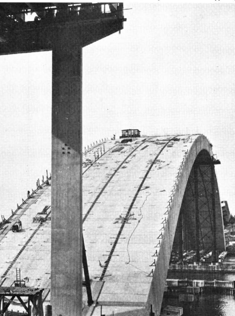
hence the overall length of the arch along its centre line. This caused it to rise and lift off the falsework making it self-supporting. The falsework was then moved sideways to carry the components of the next rib.
