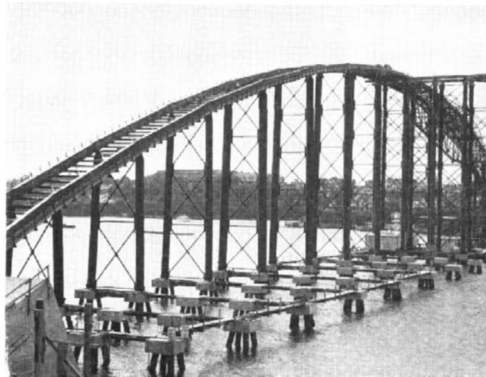
Falsework completed and ready to support the arch units
