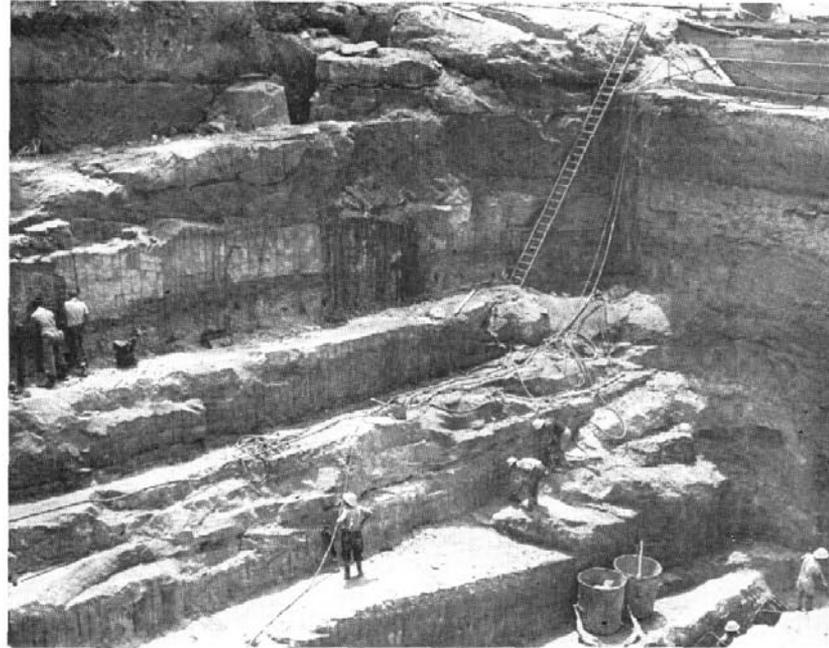
Excavation for the arch thrust blocks on the Gladesville side
