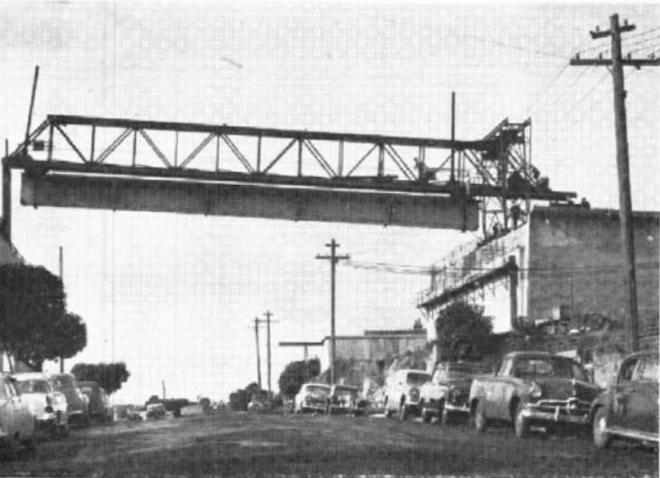
A deck beam being launched into position
