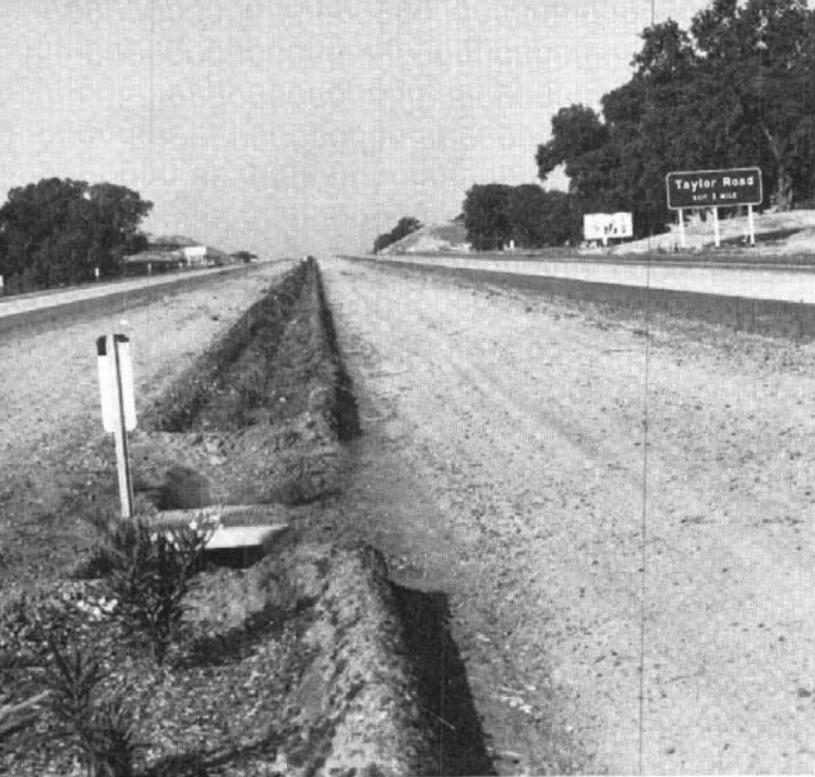
2. Wide depressed median on Interstate Route in California, U.S.A., provides favourable conditions for growing oleanders down the centre
