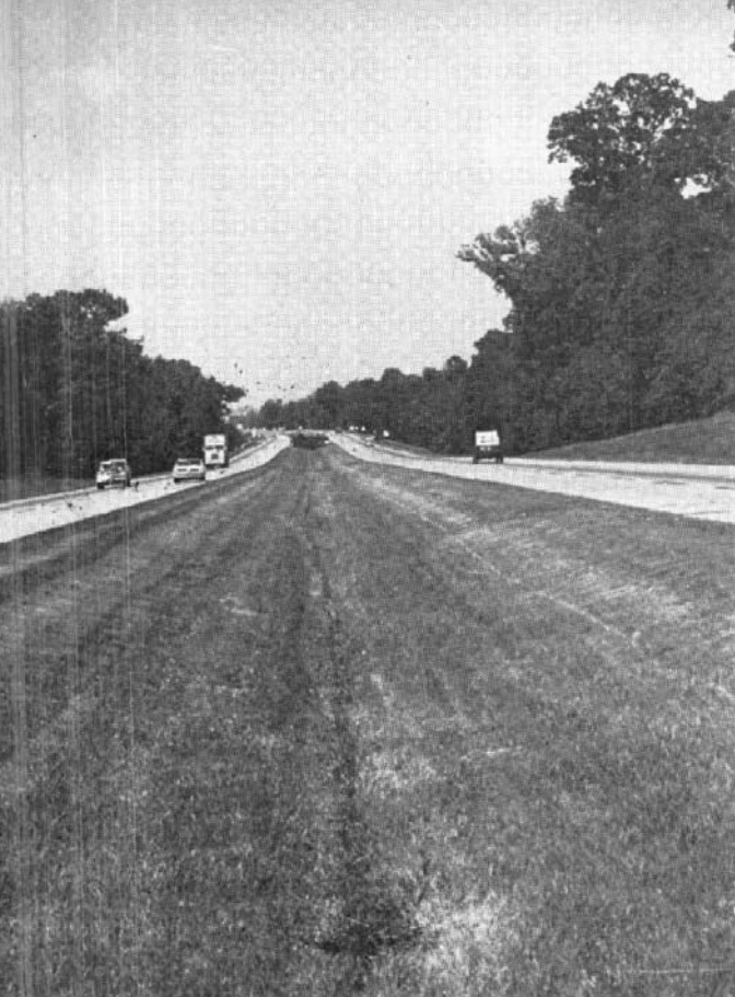
1. Depressed median on Interstate route in Illinois, U.S.A., provides for surface water disposal and acts as a barrier between two carriageways
