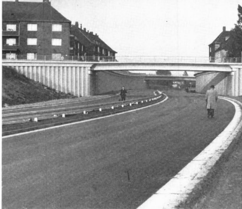
14. Urban expressway under construction in Germany shows treatment of retaining walls using sheet steel piling. The troughs of steel sheet are painted dark blue
