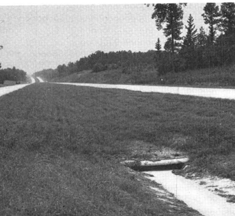
3. A grassed depressed type of median on Interstate Route in California, U.S.A., with a paved invert for drainage
