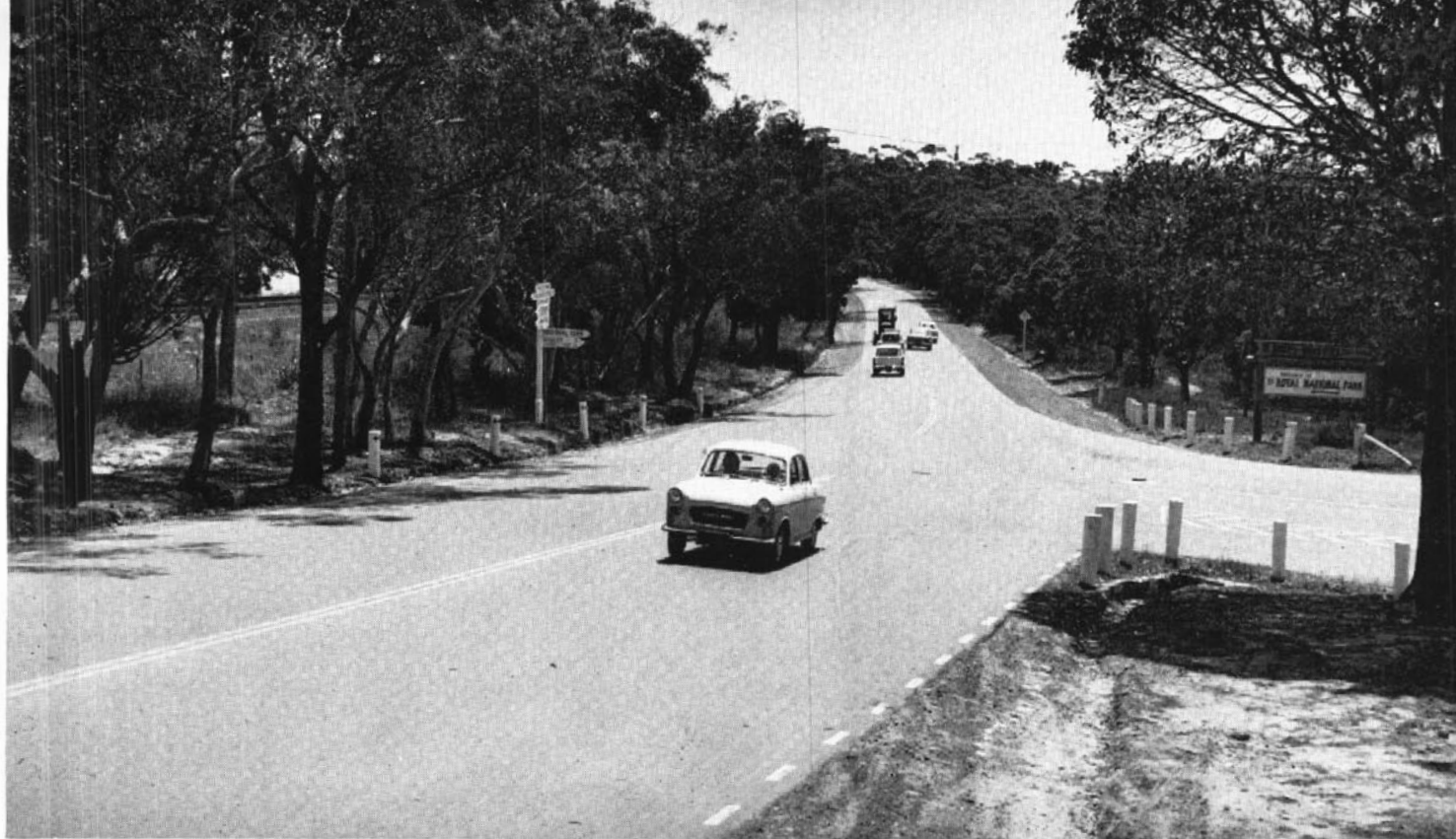
The intersection of Prince's Highway and Farnell Drive showing widening on the inside of the curve and pavement edge marking
