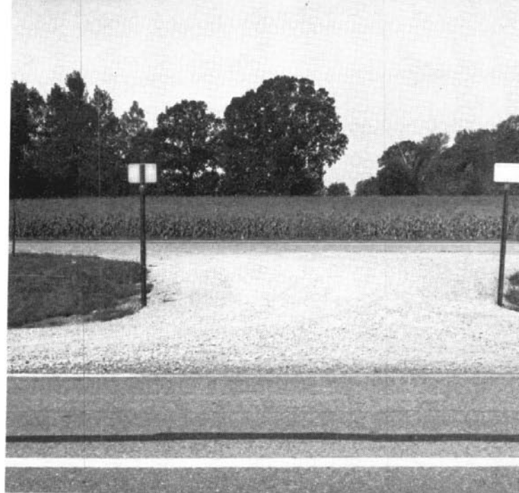
9. Emergency crossover in Ohio, U.S.A., paved with gravel. Signs read "Emergency Use Only"
