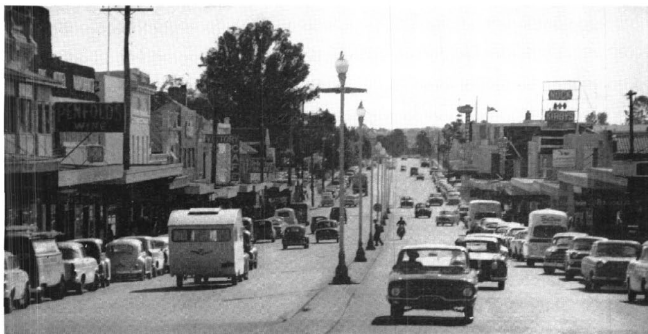
The kerbside lanes of this widened Main Road in a suburb of the Sydney Metropolitan area are being obstructed by standing vehicles, with the result that the full width of the carriageway is not available for the movement of vehicles
