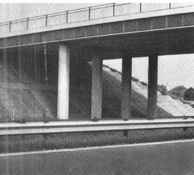
14. Urban expressway under construction in Germany shows treatment of retaining walls using sheet steel piling. The troughs of steel sheet are painted dark blue
