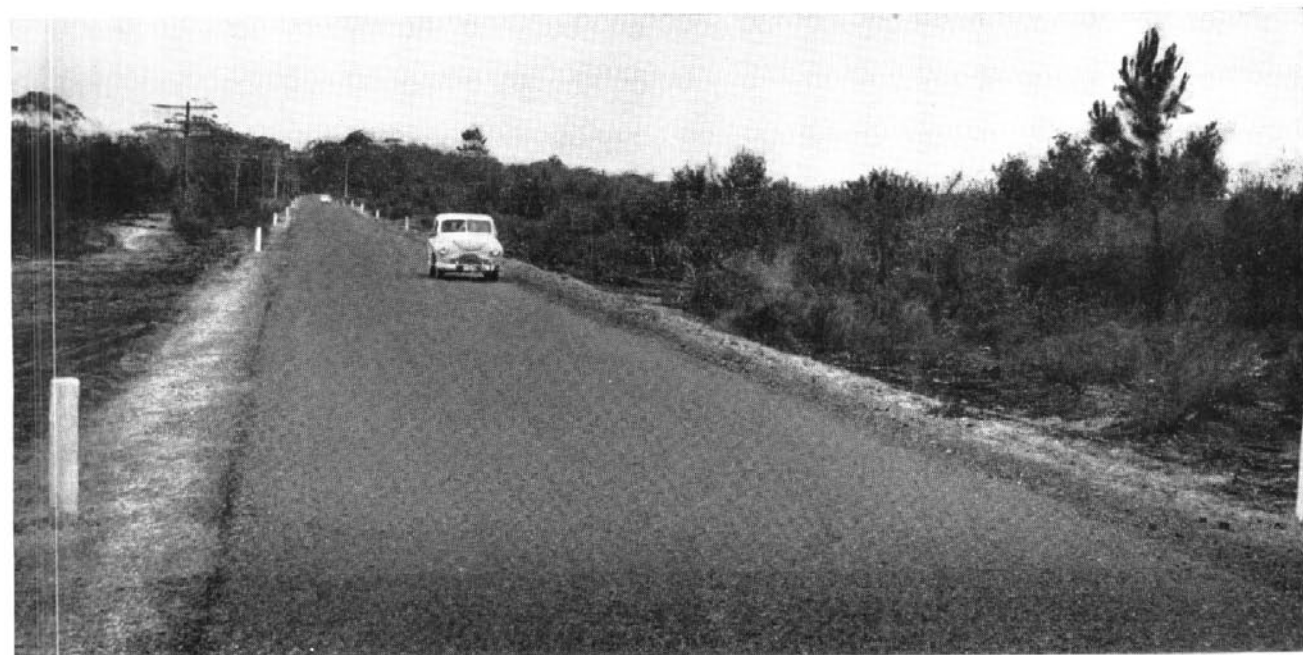
Reconstruction and bitumen surfacing carried out by the Manning Shire Council on the Tuncurry-Taree Main Road.
