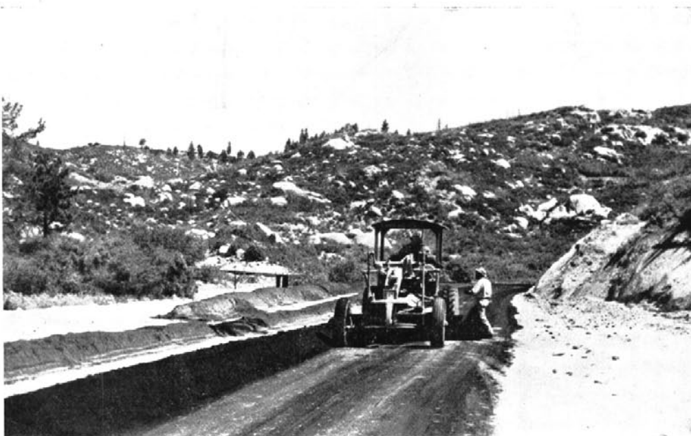
Southern California. Park road near Idyllwild. Spreading (and aerating) cold mix by power grader. After rolling, thickness of finished cold-mix course is 3 inches
