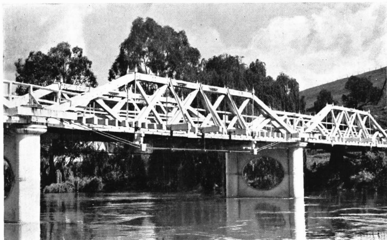
Timber Truss Bridge over Murray River at Jingellic (T.R. 85). Built in 1892 by Public Works Department. Centre Span (90 feet long) has been undertrussed.
