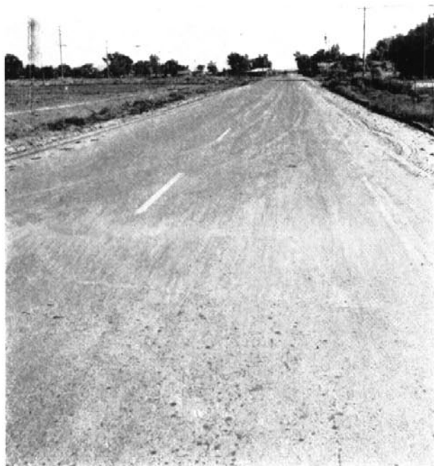
Arizona, Yuma area. View of sealed dune sand-asphalt pavement on sand formation.
