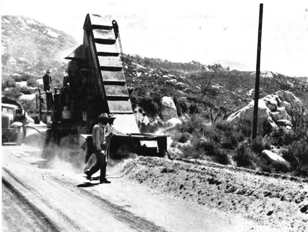
Southern California. Road in forest park at 5,000 ft. elevation near Idyllwild. Travelling continuous mixer for production of cold mix from local decomposed granite gravel and 6.6% of S.C. 3 asphaltic binder. Output is 1,250 tons in 8 hours.
