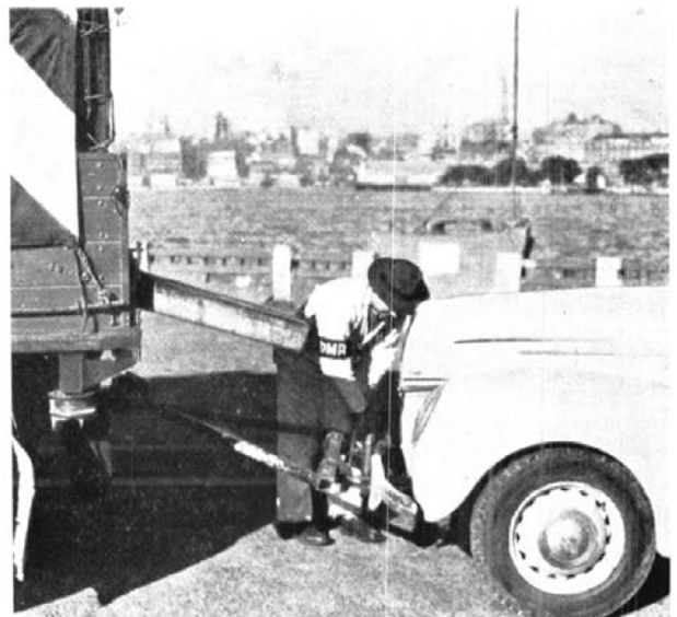
Method used for bumper-bar Tow.
