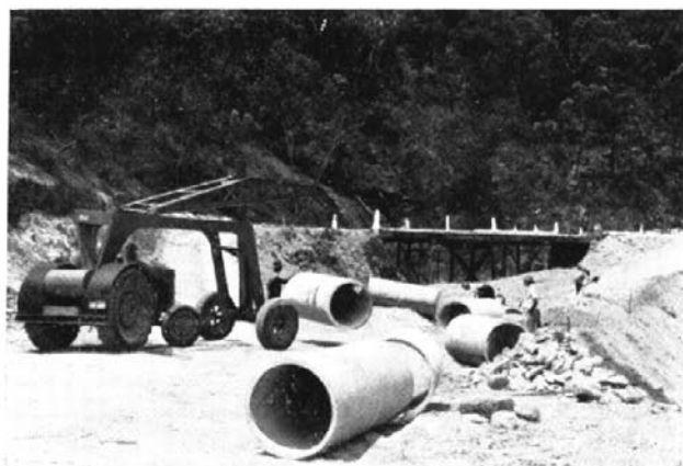
Concrete Pipes being lifted into position.
