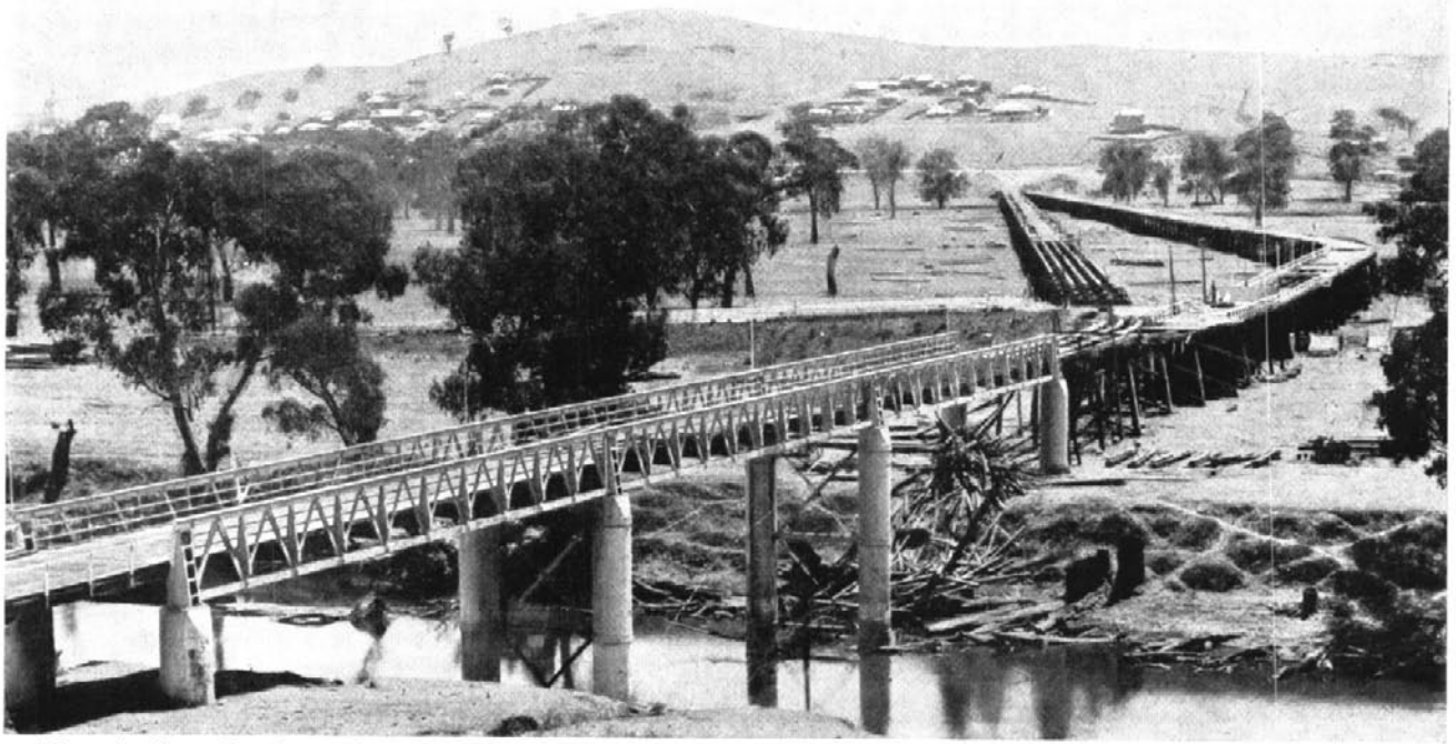
Wrought Iron Continuous Truss Bridge over Murrumbidgee River, Gundagai (Hume Highway). Built in 1866 by Public Works Department. Photo taken in 1896 when old timber approach spans were rebuilt.
