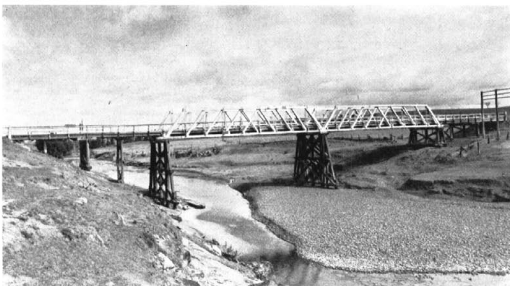
Timber Truss Bridge over Glennie's Creek north of Singleton, New England Highway. Built in 1895 by Public Works Department. Length of spans, 90 feet.
