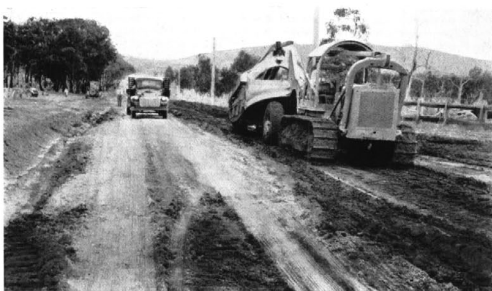
80 H.P. Tractor with 8 cub. yd. Scoop at work.
