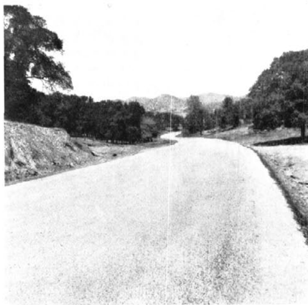
California, Tuolumne County. Newly completed secondary road with sealed shale pavement.
