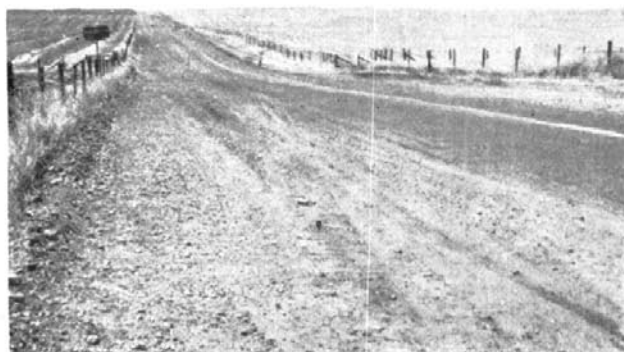
California. S.H. 41 near Fresno. Low cost "oiled" surface.
