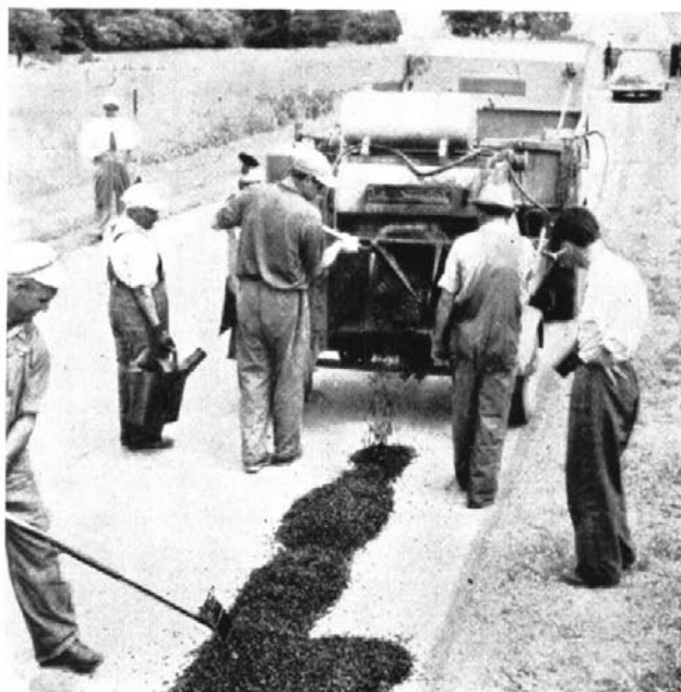
Ohio, Knox County. Improvised mobile unit for production of semi-hot mix for maintenance purposes. View is of concrete mixer drawn behind maintenance truck carrying aggregate.
