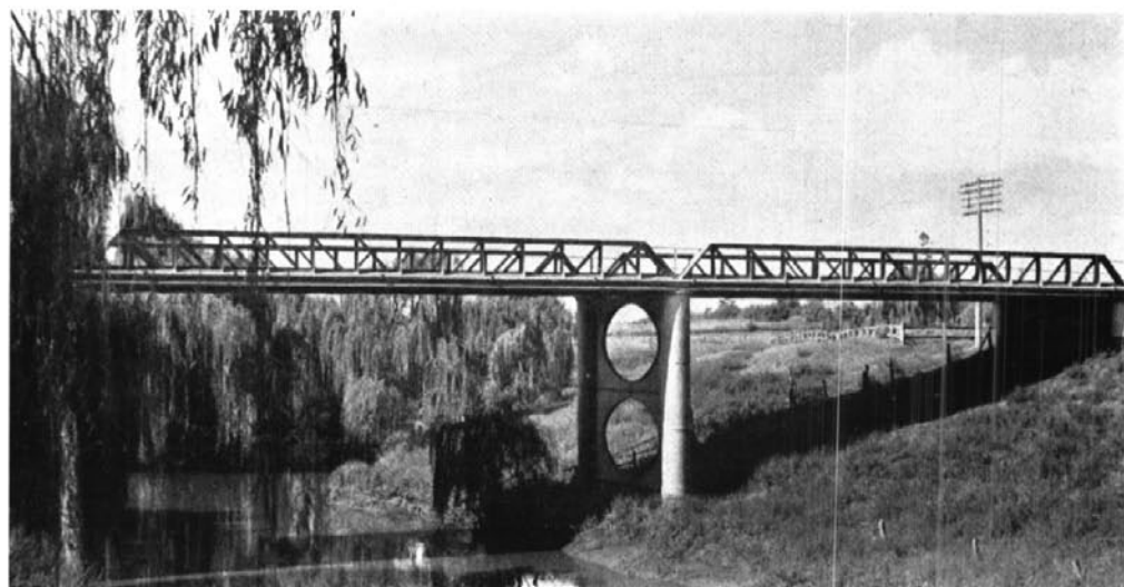
Wrought Iron Truss Bridge over South Creek, Windsor (M.R. 184). Built in 1879 by Public Works Department.
