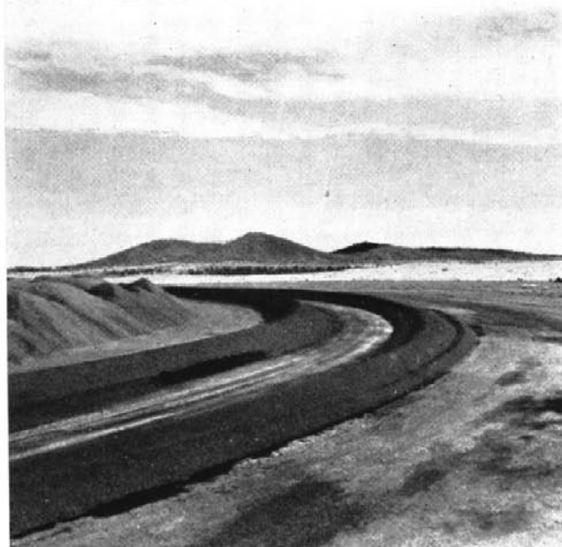
Arizona. Roadside production of maintenance cold-mix. Outer circular windrow is of finally mixed materials.
