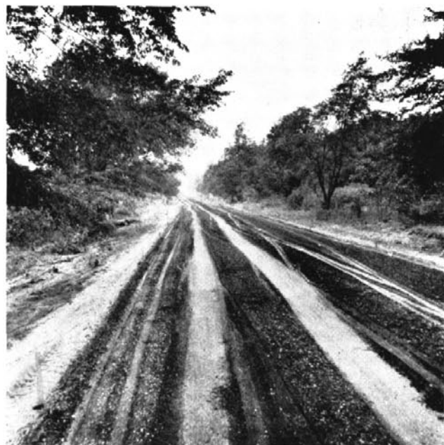
Oceana County, Michigan. Experimental length of gravel mixed with sand—formation using asphaltic binder. View after second application, mixing and spreading.
