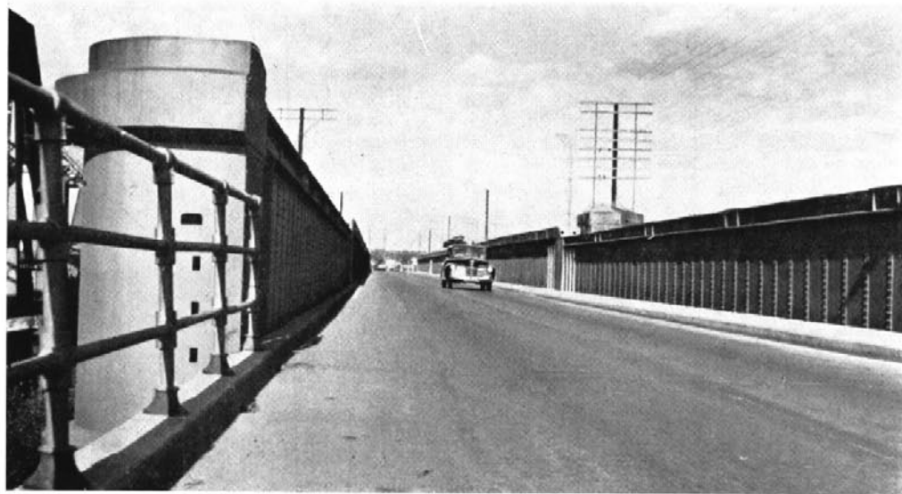
Wrought Iron Box Girder Bridge Built in 1897 over Nepean River, Penrith, Great Western Highway. Originally carried Railway but converted to road use in 1907.
