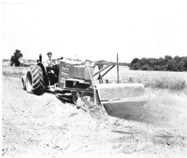
North Carolina. Mixing clay with sand soil to produce a 6 inch base to carry a sand-asphalt running course.
