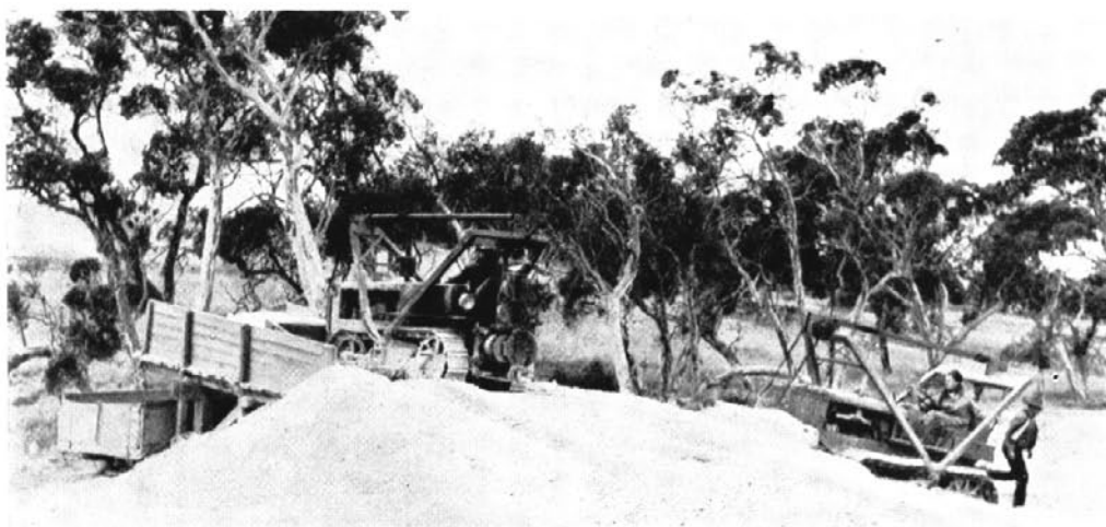
Tractors bringing in and loading gravel into truck through side loader.
