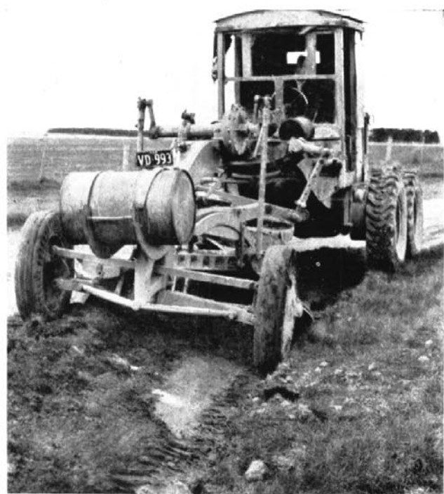
Heavy Duty Motor Grader cutting outlet from Table Drain.
