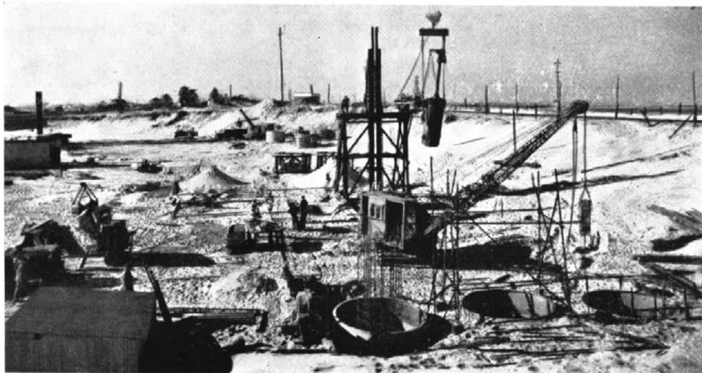
Bridge foundations under construction in partly excavated channel.
