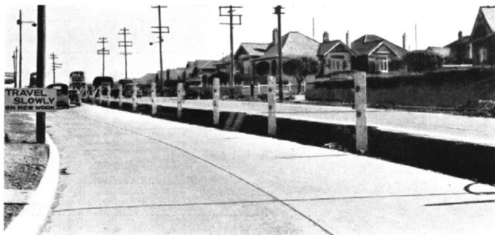
View showing difference in levels between new and old pave- ments.
