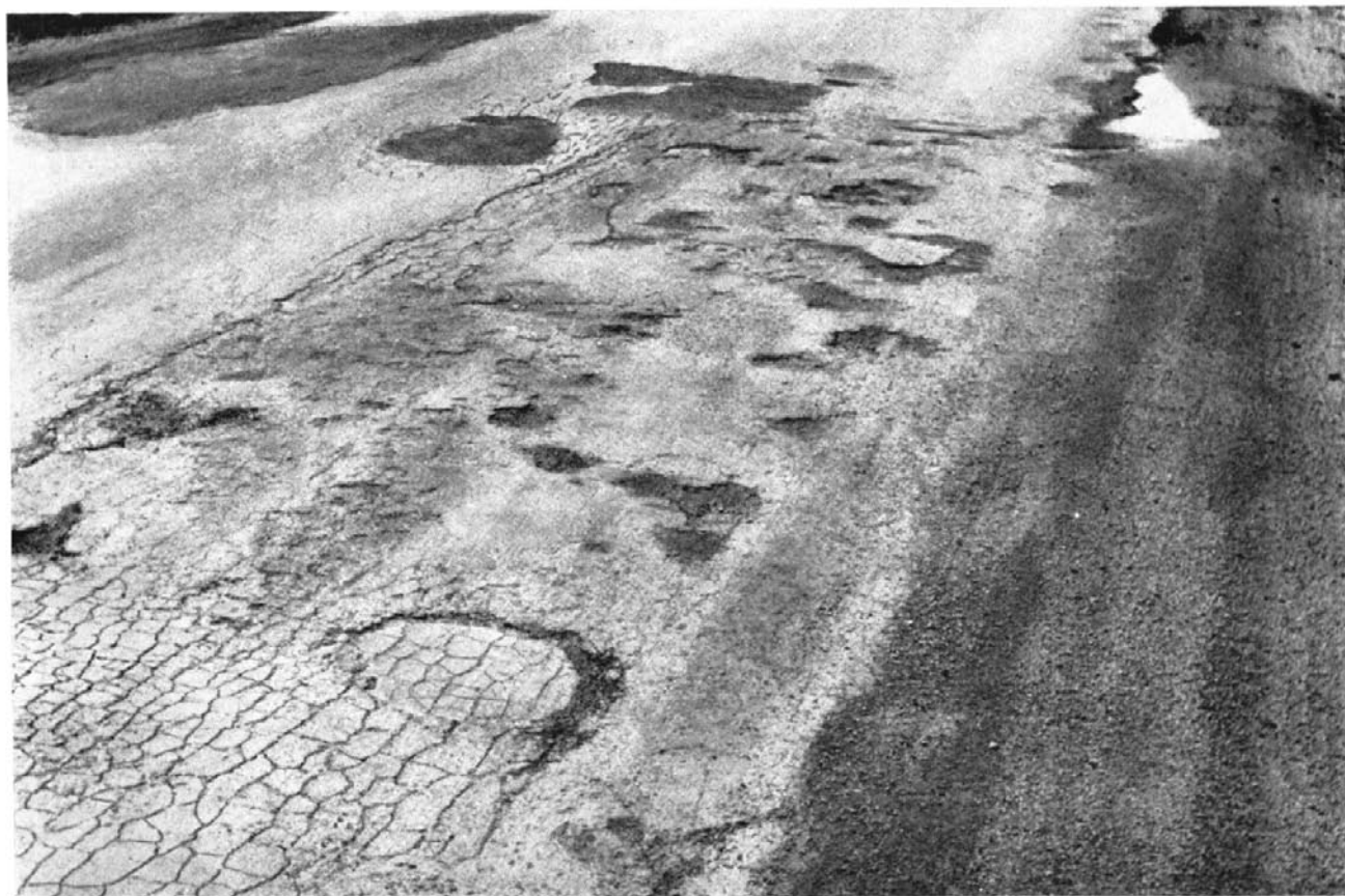
Example of pavement failure on Hume Highway on Breadalbane Plains between Goulburn and Gunning.
