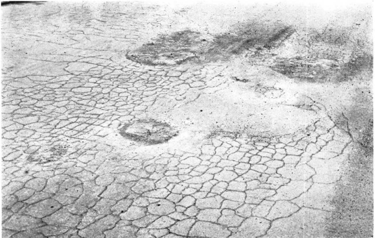
Pavement failure on Great Western Highway on the Blue Mountains.
