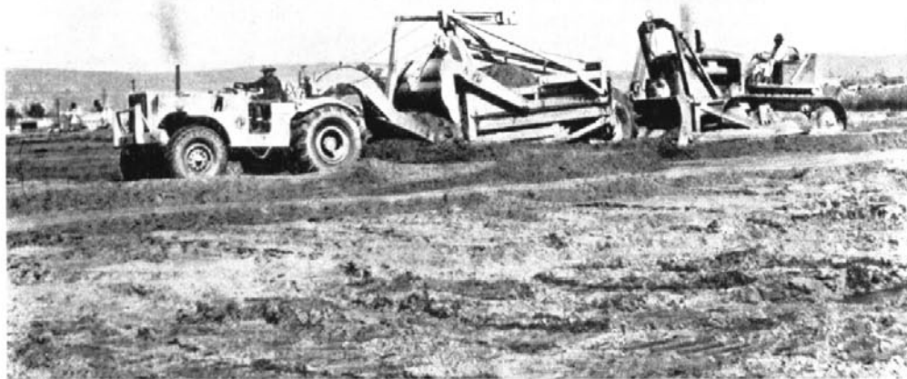
Four-wheeled Tractor and 12 cu. yd. scoop used for earth movement on long leads. Bulldozer used to assist loading.
