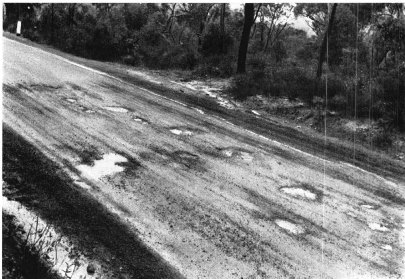
Typical pavement failure on the Pacific Highway between Peat's Ferry and Gosford.
