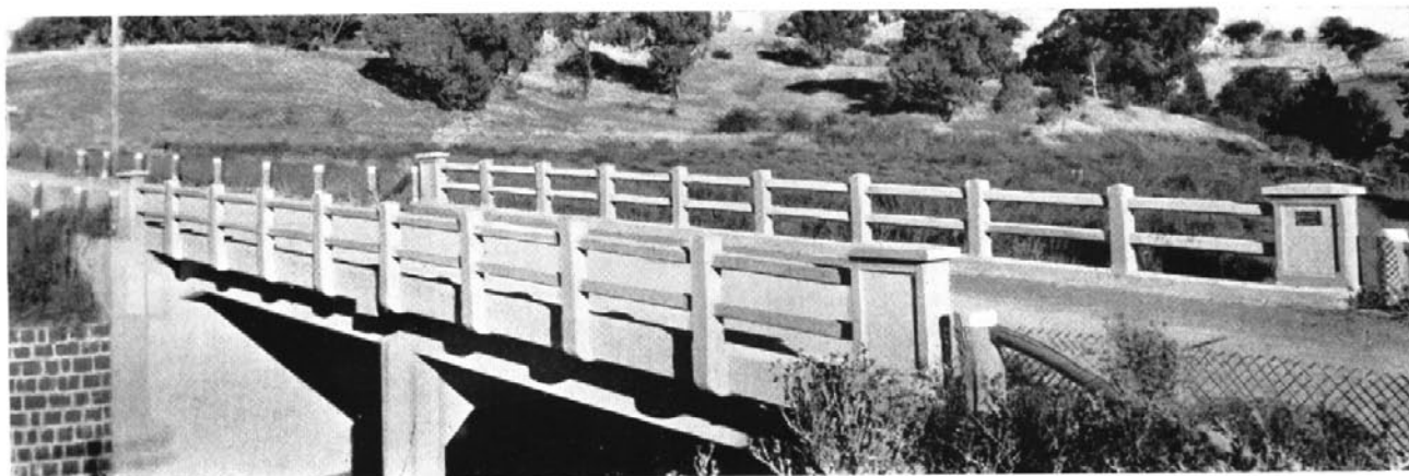
Fig. 2. Reinforced concrete posts and rails.
