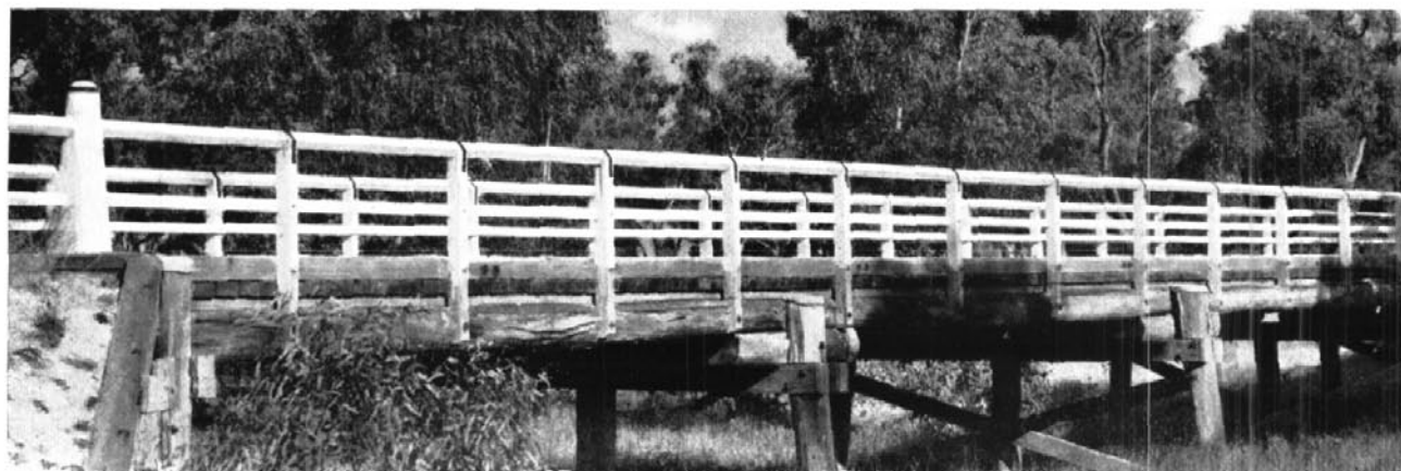
Fig. 14. Timber posts and rails on typical timber beam bridge.
