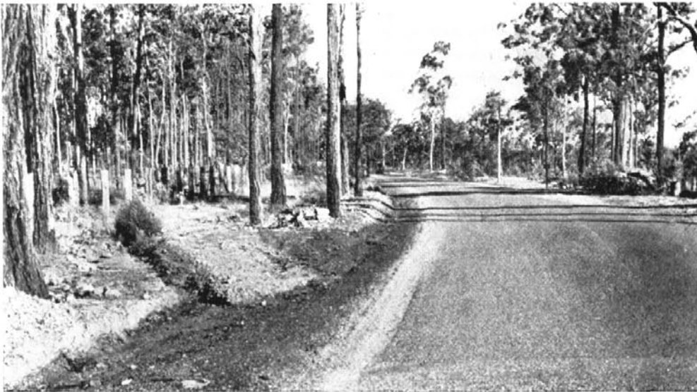
Illustrating a case where water is wrongly being discharged from the catch drain to the table drain, overloading the table drain, and creating liability to scour. The catch drain should have been continued behind the trees on left to discharge to a nearby watercourse.
