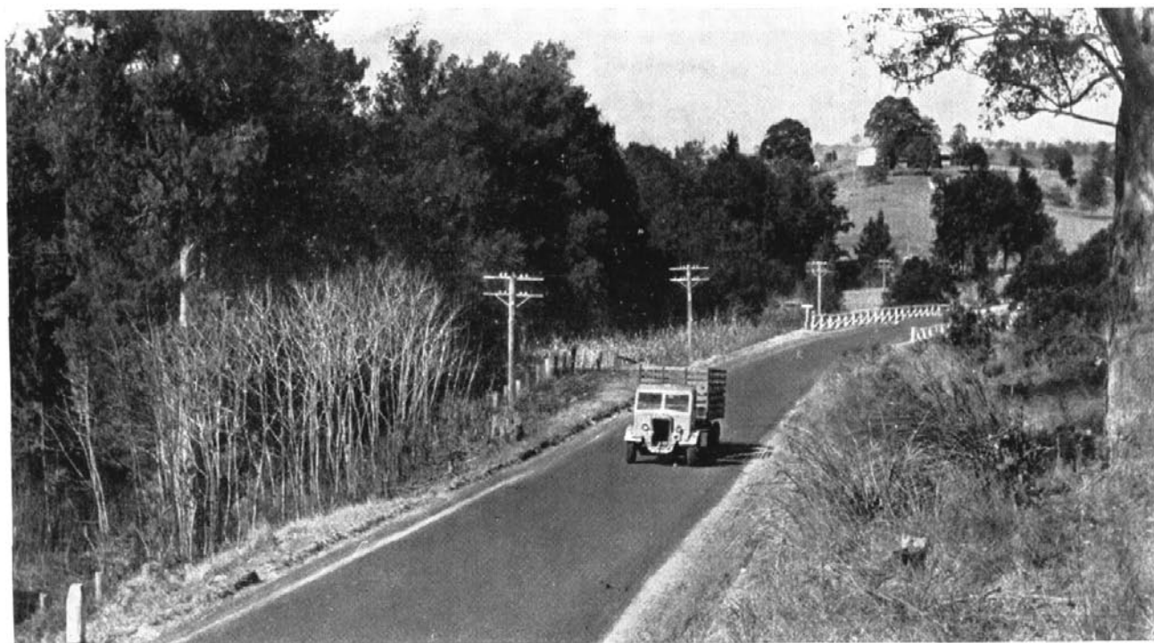
A section of Prince's Highway between Brogo River and Allsop's Creek near Bega after construction and bituminous surfacing.
