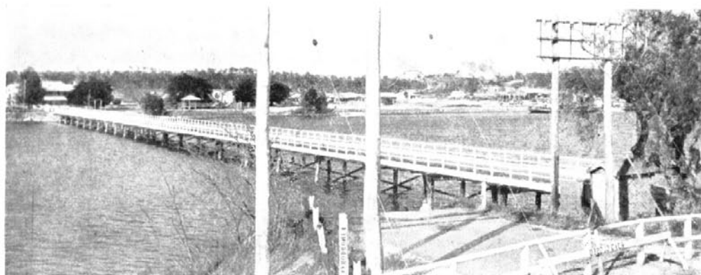
Temporary Rolled Steel Joist Bridge with Timber Deck over Moruya River, built to replace old bridge destroyed by flood.
