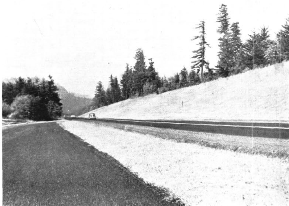
Four-lane divided highway with depressed median and flattened slopes in cutting. Median and sides of cuttings are grassed.
