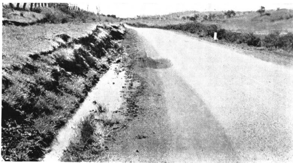
Failure of a patch owing to the cause of original failure having been neglected
