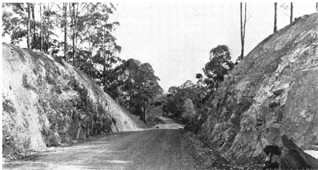
Reconstructed section of Pacific Highway, 3 m. from Coff's Harbour, showing heavy earthworks.
