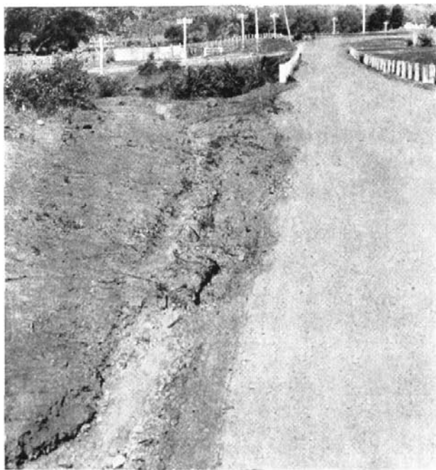
Damage caused by scouring because table drain and entrance to side drains were blocked when pavement was graded.
