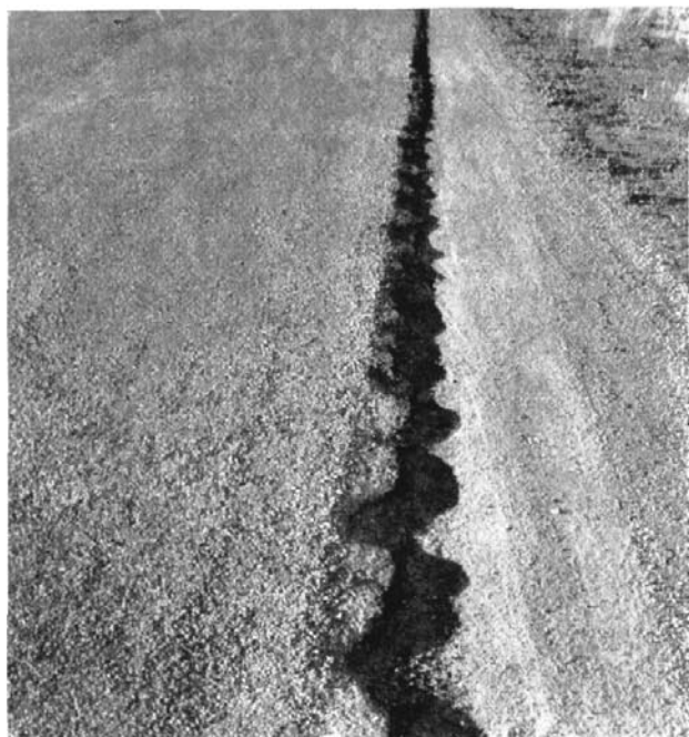
Typical case of reduction in width of a "black top" pavement caused through neglect to maintain edges.
