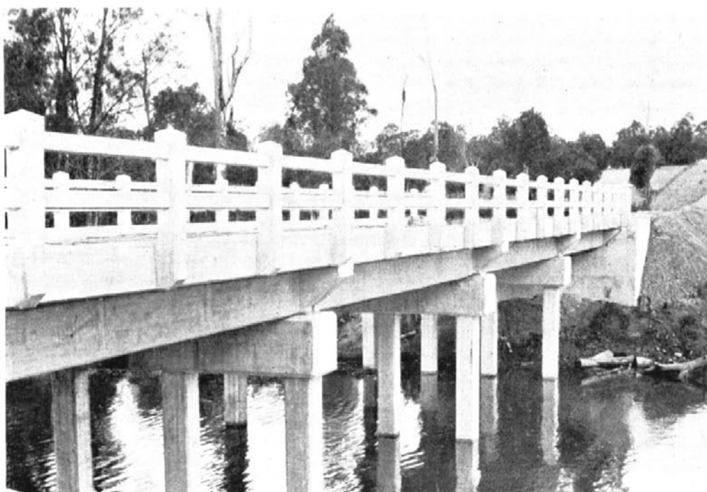
New reinforced concrete bridge on concrete piles over Middle Boambee Creek.
