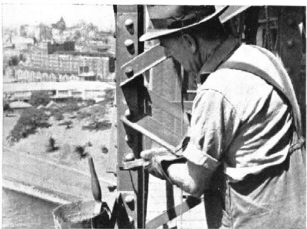
Scraping and painting of Under Span Gantry.
