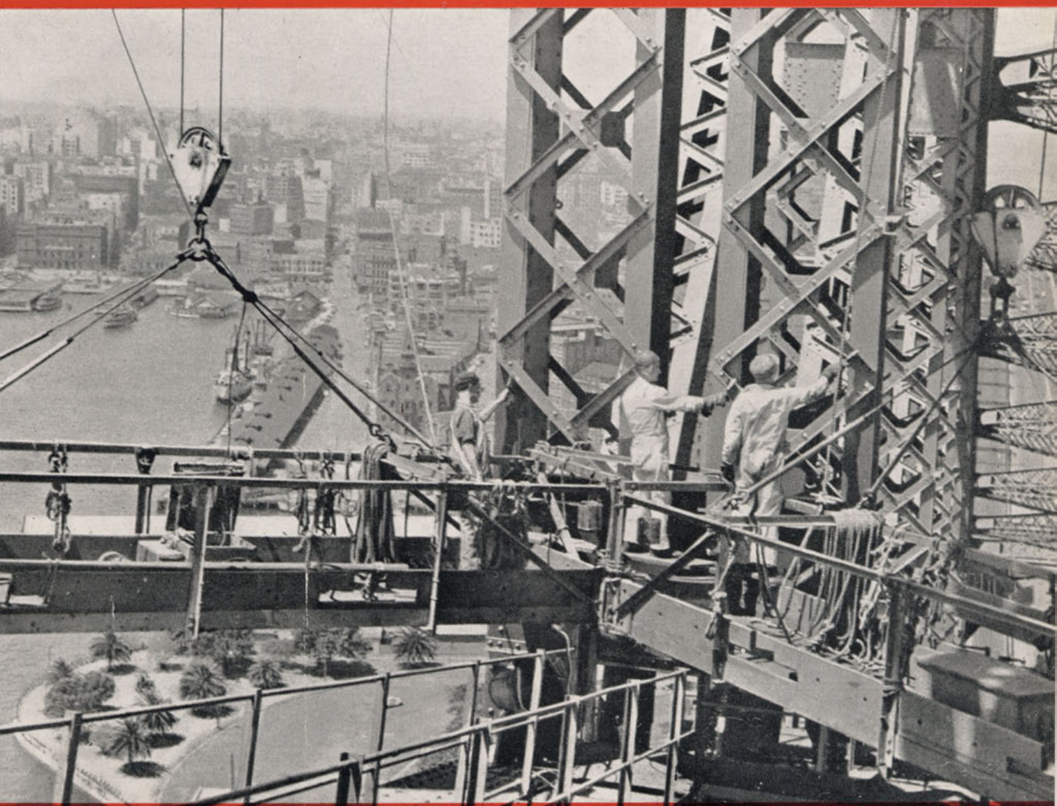
Painting members of the Main Arch Span, Sydney Harbour Bridge. Painters working from stages suspended from cranes situated on top of arch. Circular Quay, Sydney, can be seen to the left.
