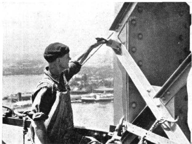
Painter working off Crane Stage.
