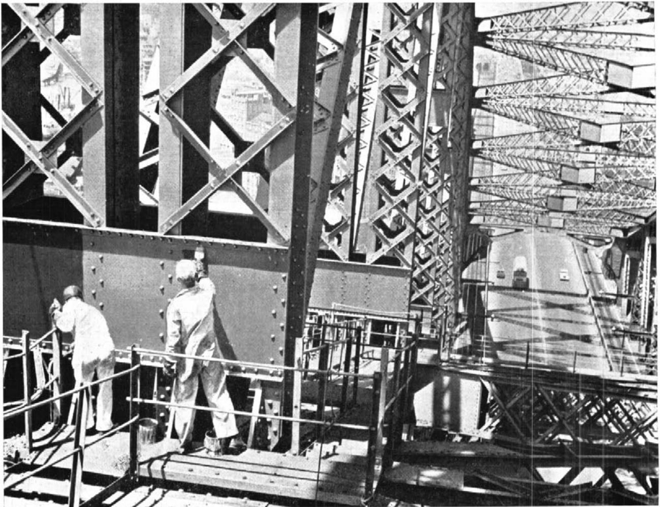
Painters working from Lower Chord of Main Span.
