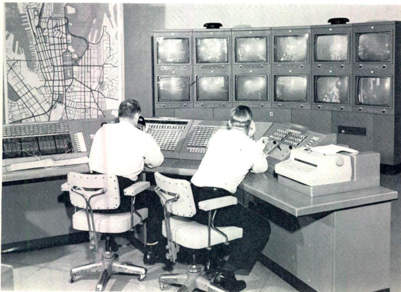
Supervision and control of the Inner-City signal complex is maintained from a central control room (pictured below) where the traffic flow is monitored by the use of twelve cameras, each with a separate screen. One phase of the signalling at the intersection illustrated in the upper picture allows pedestrians complete use of the crossing facilities whilst all traffic is halted.
