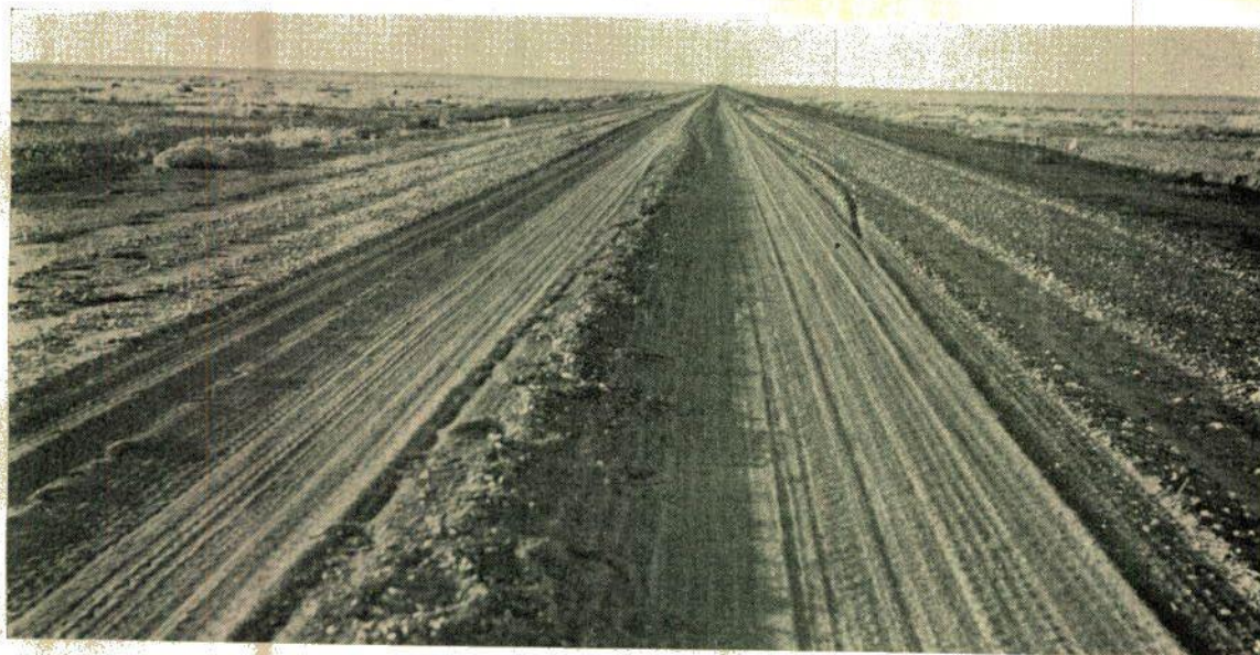
State Highway No. 22. Broken Hill-Tibooburra-road. New formation as yet unconsolidated.
