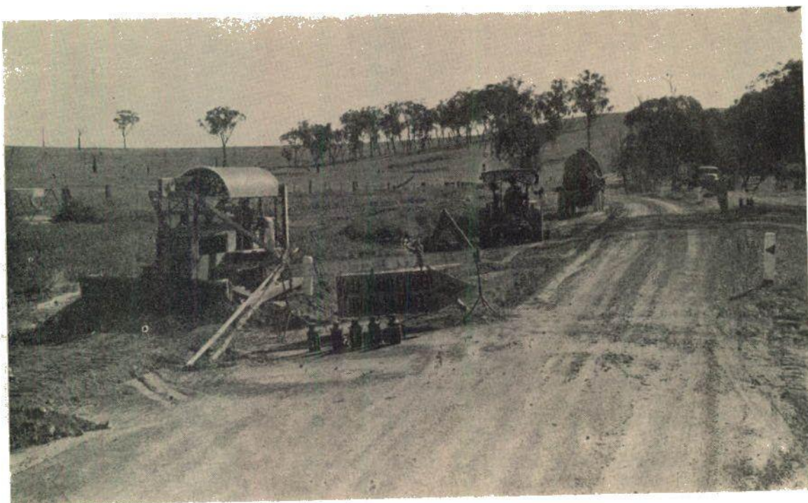
Hume Highway. Repairing damage following recent growth of long-distance heavy haulage. (Shire of Gundagai.)
