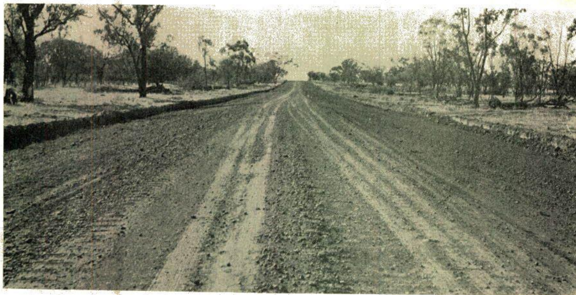
State Highway No. 18. Walgett to Queensland border. New formation constructed by elevating grader north of Angledool.
