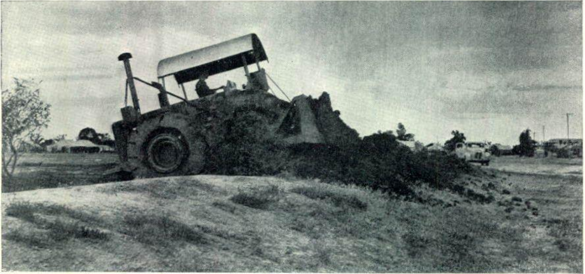
132-h.p. pneumatic-tyred tractor dozer diverted from road work to assist Wentworth Municipal Council, strengthening levee banks to withstand flooding from Darling River.
