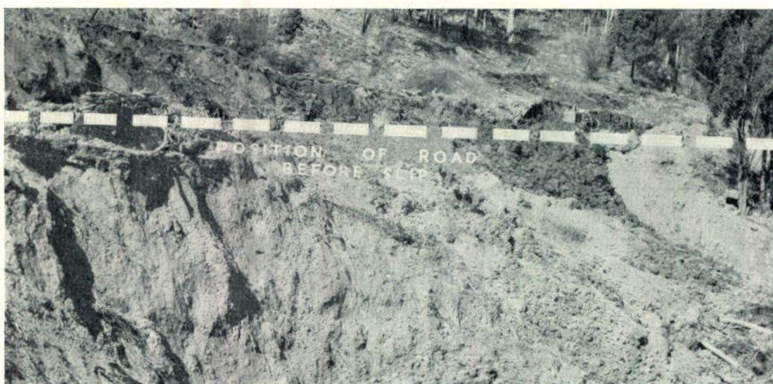
Collapse of section of Hume Highway (S.H. 2), on Razorback Range, between Camden and Picton, as a result of landslides. Shire of Wollondilly.
