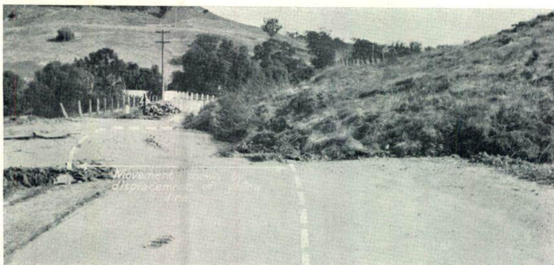
Movement of road by typical landslide. Hume Highway (S.H. 2), between Razorback Range and Picton. Shire of Wollondilly.
