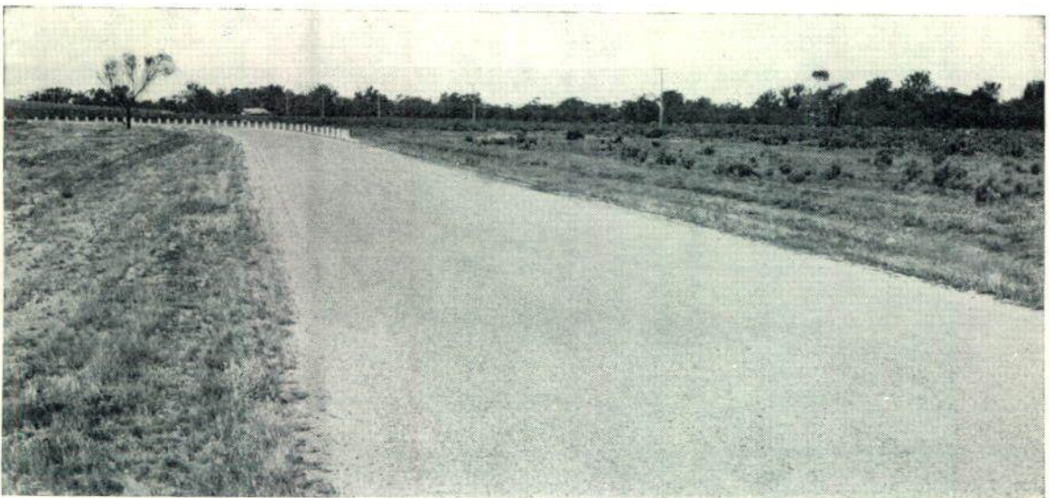
New bituminous pavement between Wentworth and Dareton (S.H. 22).
