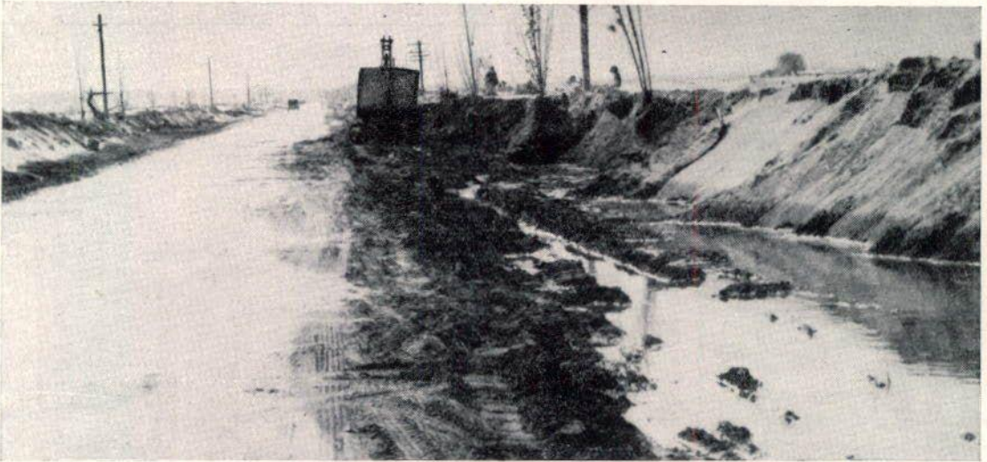
Clearing soil and silt from Pacific Highway (S.H. 10), between Kempsey and Frederickton. Shire of Macleay. During flood the road was covered with soil and silt over a length of almost a mile to a depth averaging 3 feet to 4 feet.
