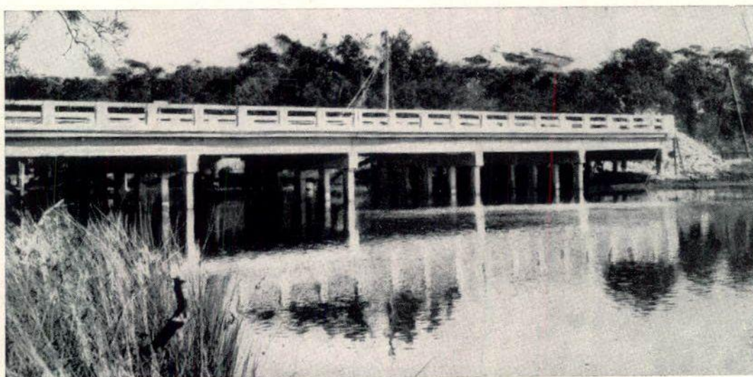
New reinforced concrete bridge over Toubouree Lake on the Prince's Highway (S.H. 1), Shire of Shoalhaven.
