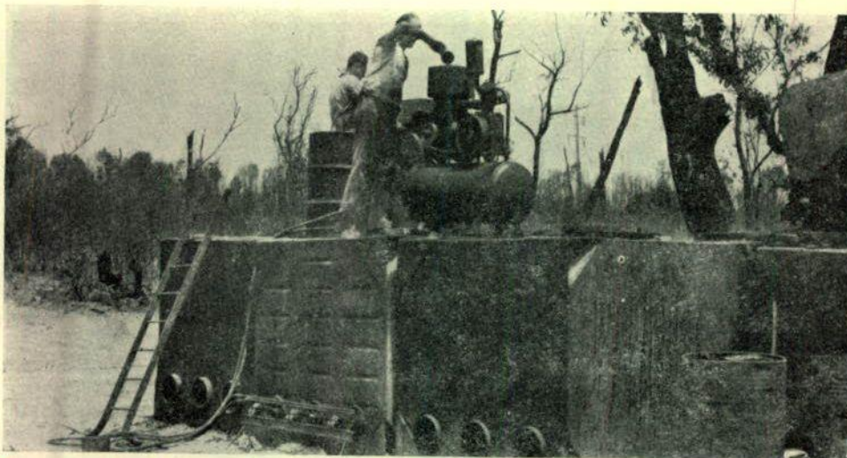
Tanks used for bitumen delivery and roadside heating. Provided by bitumen suppliers.
