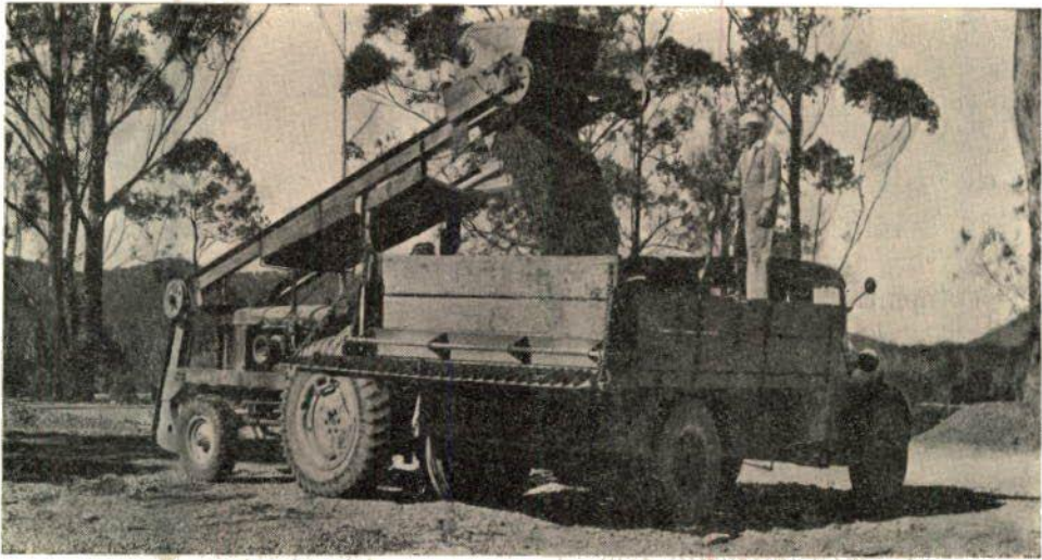
Mechanical loading of aggregate for bitumen surfacing work.
