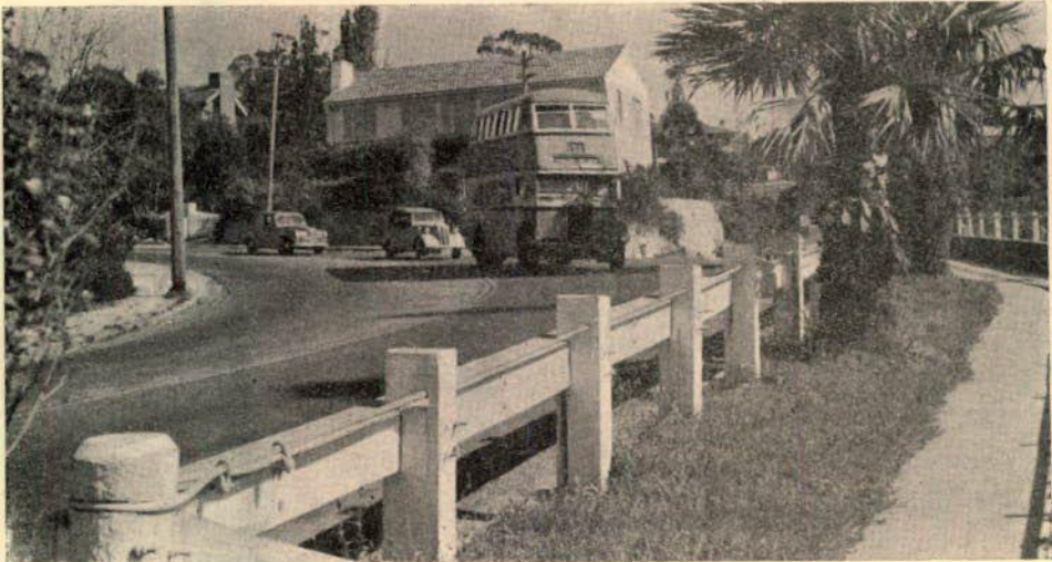
Heavy-type protection fencing as installed at some sharp bends in Metropolitan area. View on Spit Hill (M.R. 164). Municipality of Mosman.
