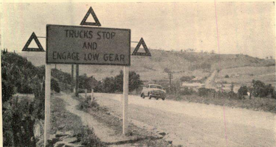
Special type warning sign as installed at approach to a steep grade followed by a sharp bend. Sign shown is at approach to subway at Picton. Hume Highway. (S.H.2.). Shire of Wollondilly.
