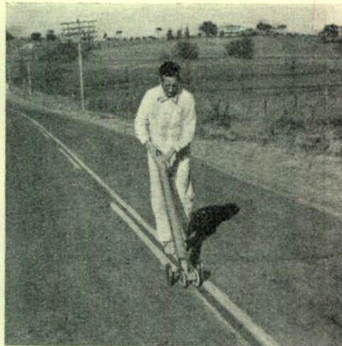
Manual line marker used for repairing traffic lines.
