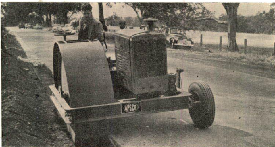
Trench roller used for pavement widening work.
