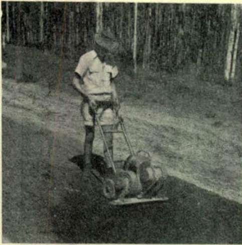
Vibrating tamper for compacting bituminous patches.
